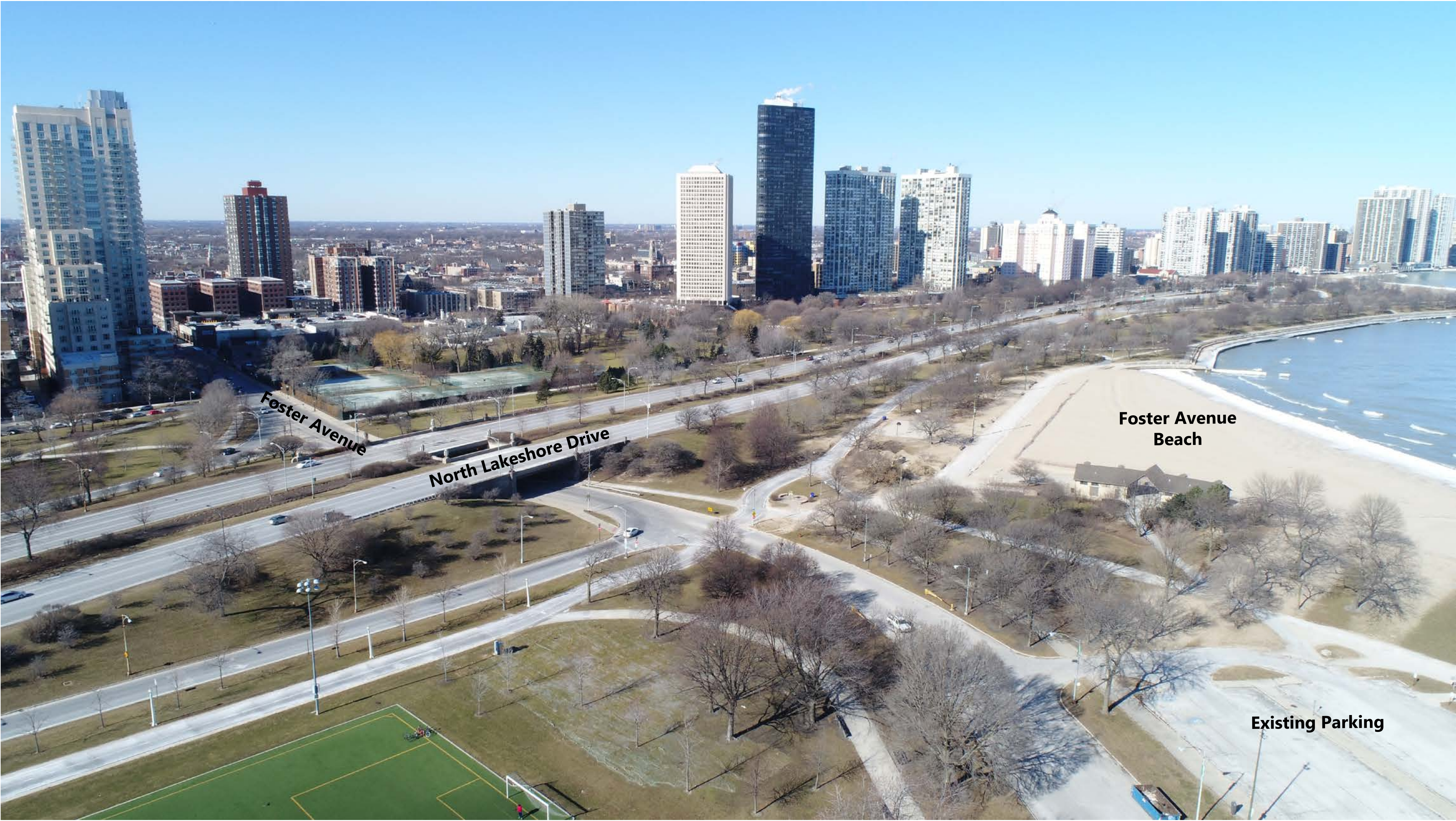
Foster Avenue, Looking North - EXISTING VIEW
