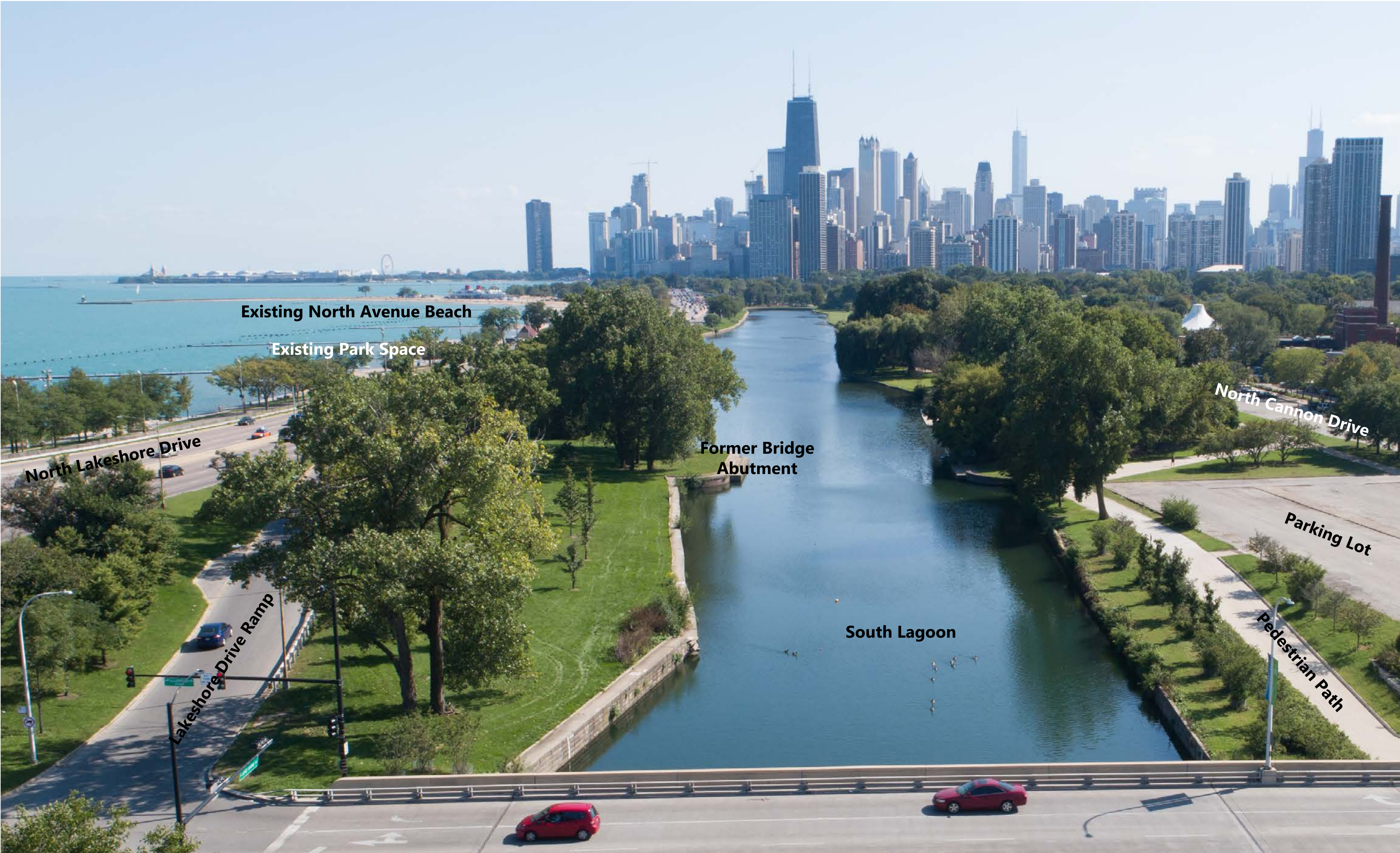
Fullerton Avenue Bridge, Looking South- EXISTING VIEW
