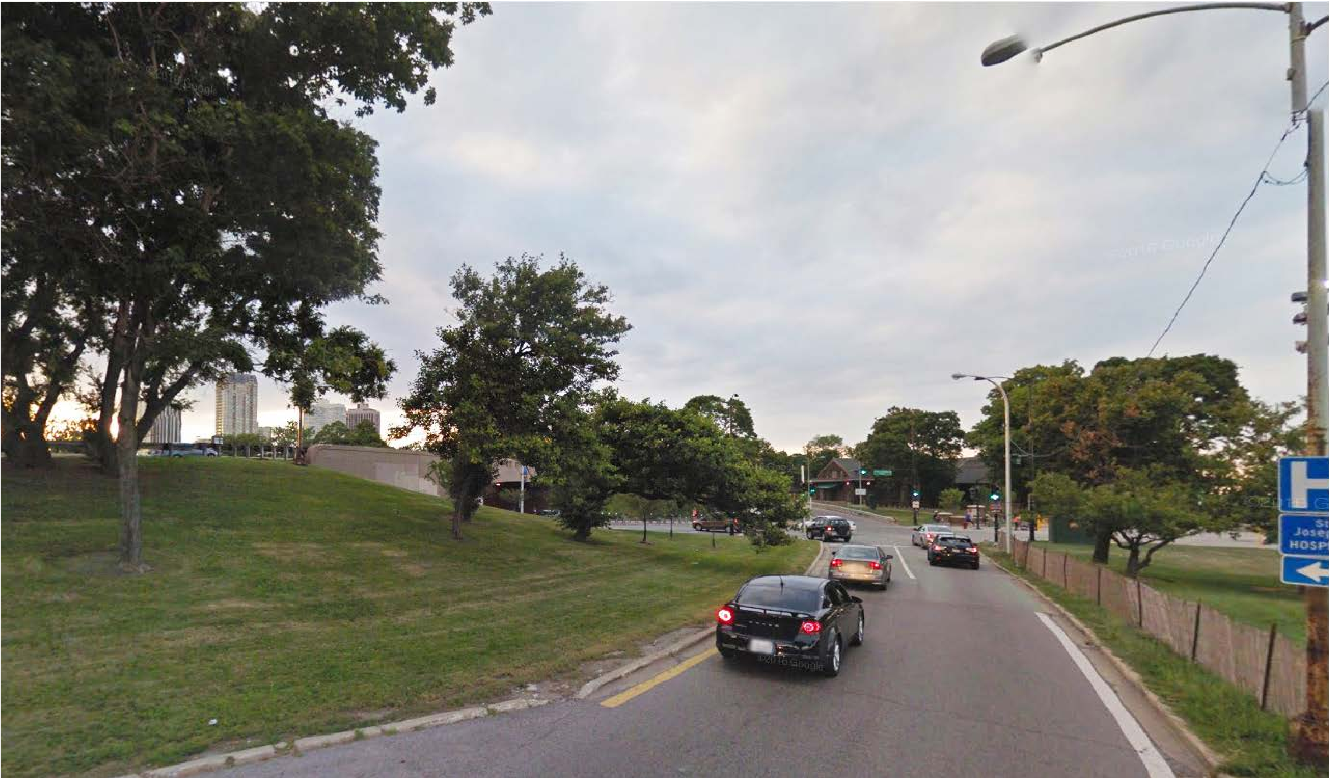
Typical Existing Junction with Grass Embankment - EXISTING VIEW
