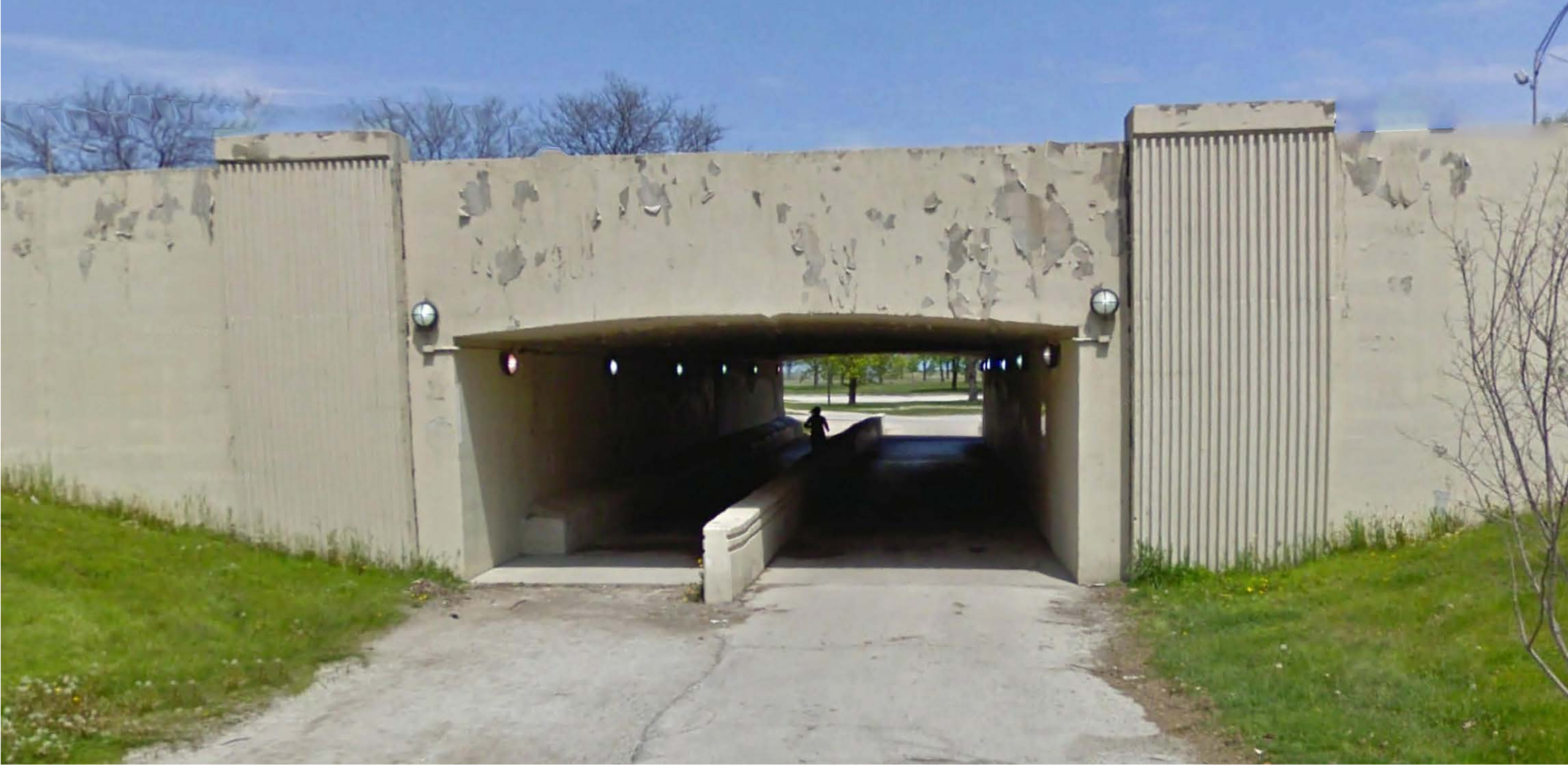
Typical Pedestrian Underpass- EXISTING VIEW
