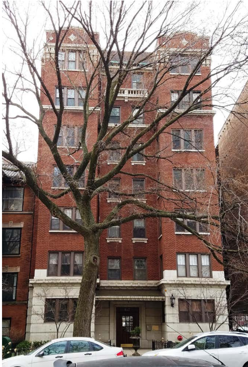
647 W. Sheridan Road, view looking south from W. Sheridan Road toward North façade
