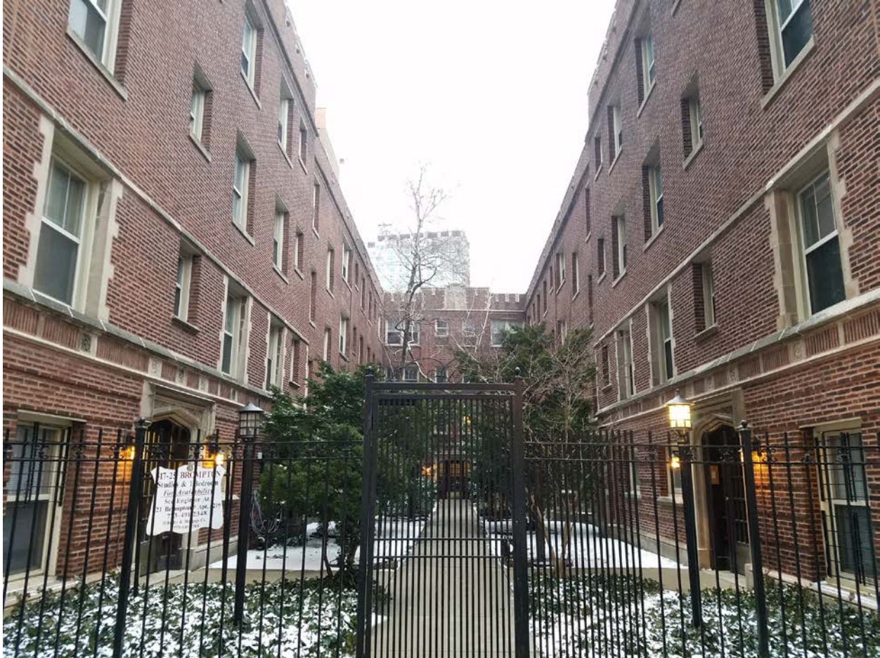
517-525 W. Brompton Avenue, view looking South from W. Brompton Avenue
