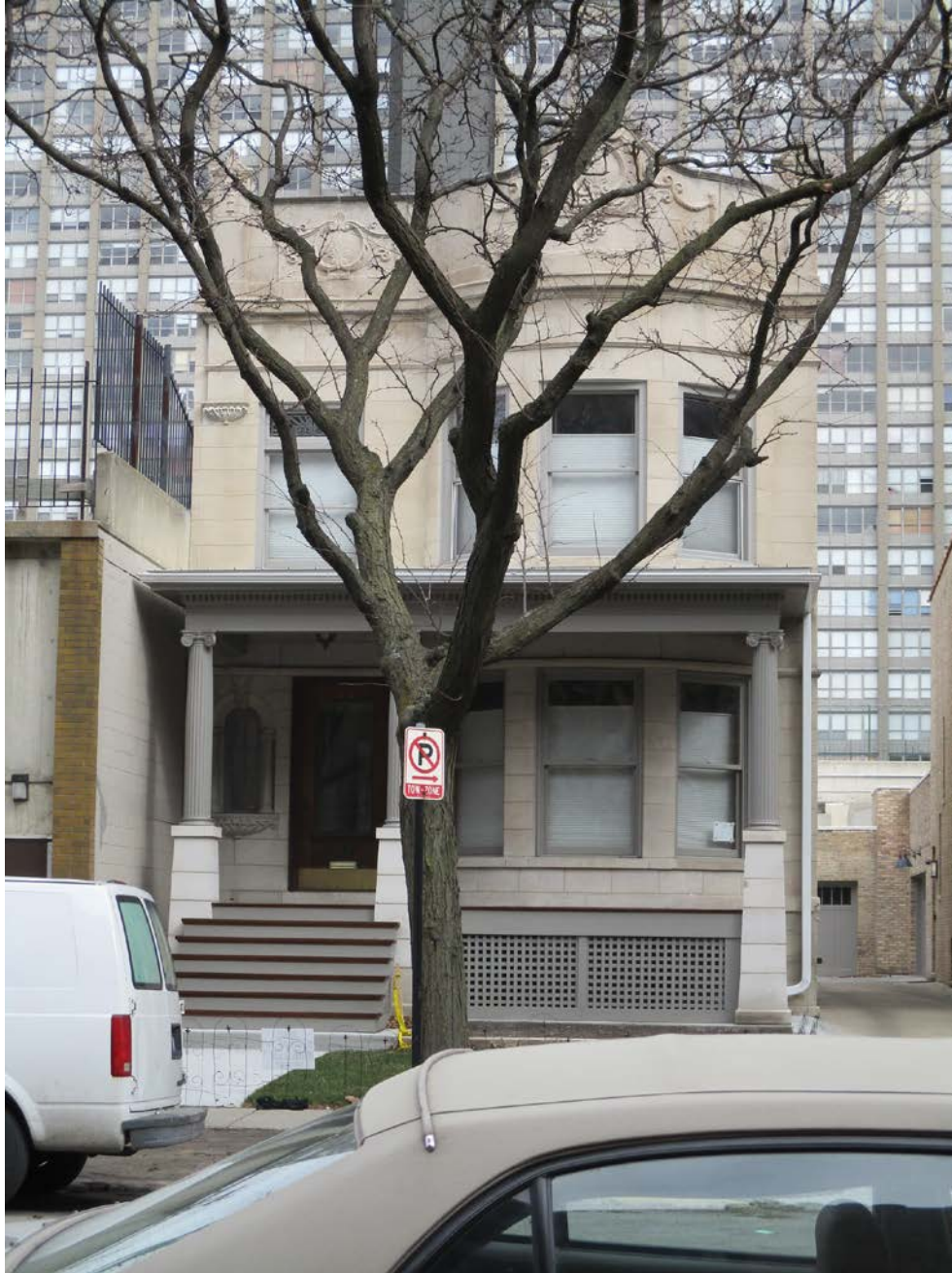
656 W. Sheridan Road, view looking north from W. Sheridan Road toward South façade
