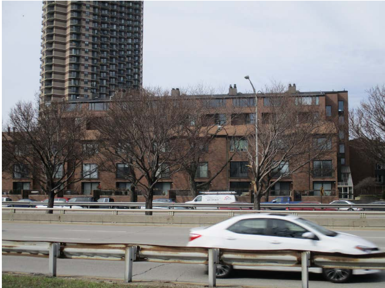
3700 N. Lake Shore Drive, view looking west from N. Lake Shore Drive toward East façades
