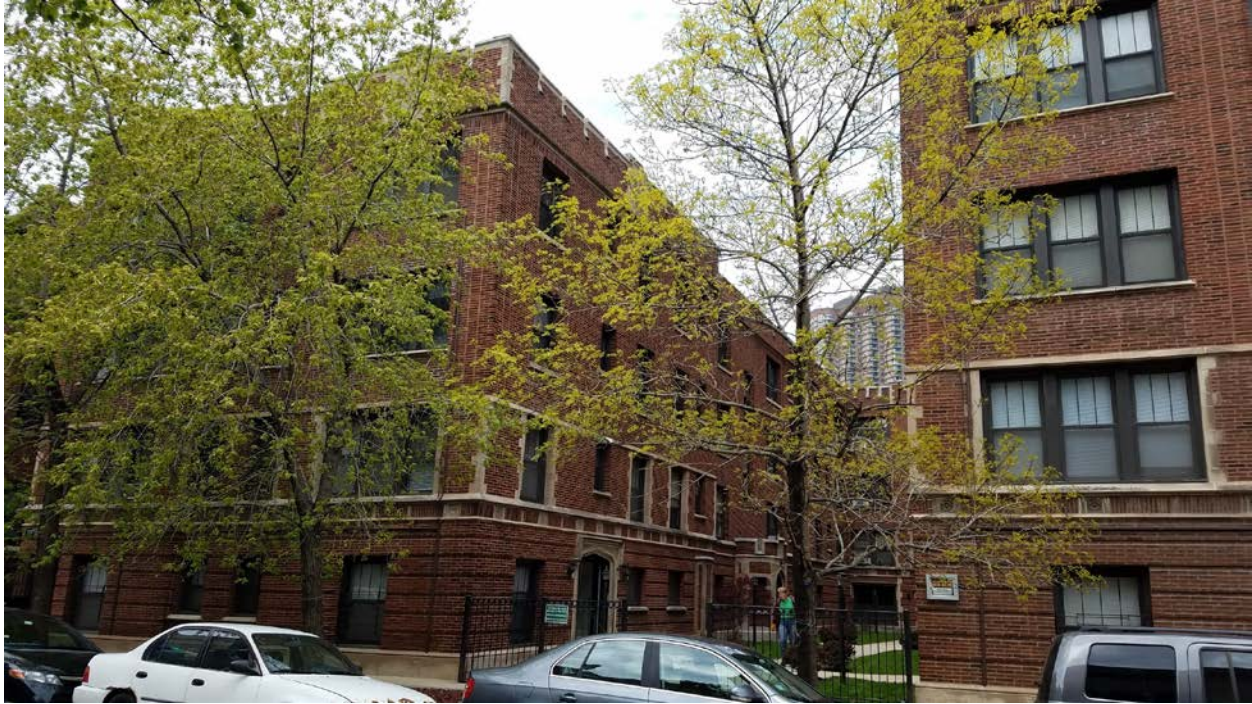
512-520 W. Cornelia Avenue, view looking northwest from W. Cornelia Avenue toward South and East façades
