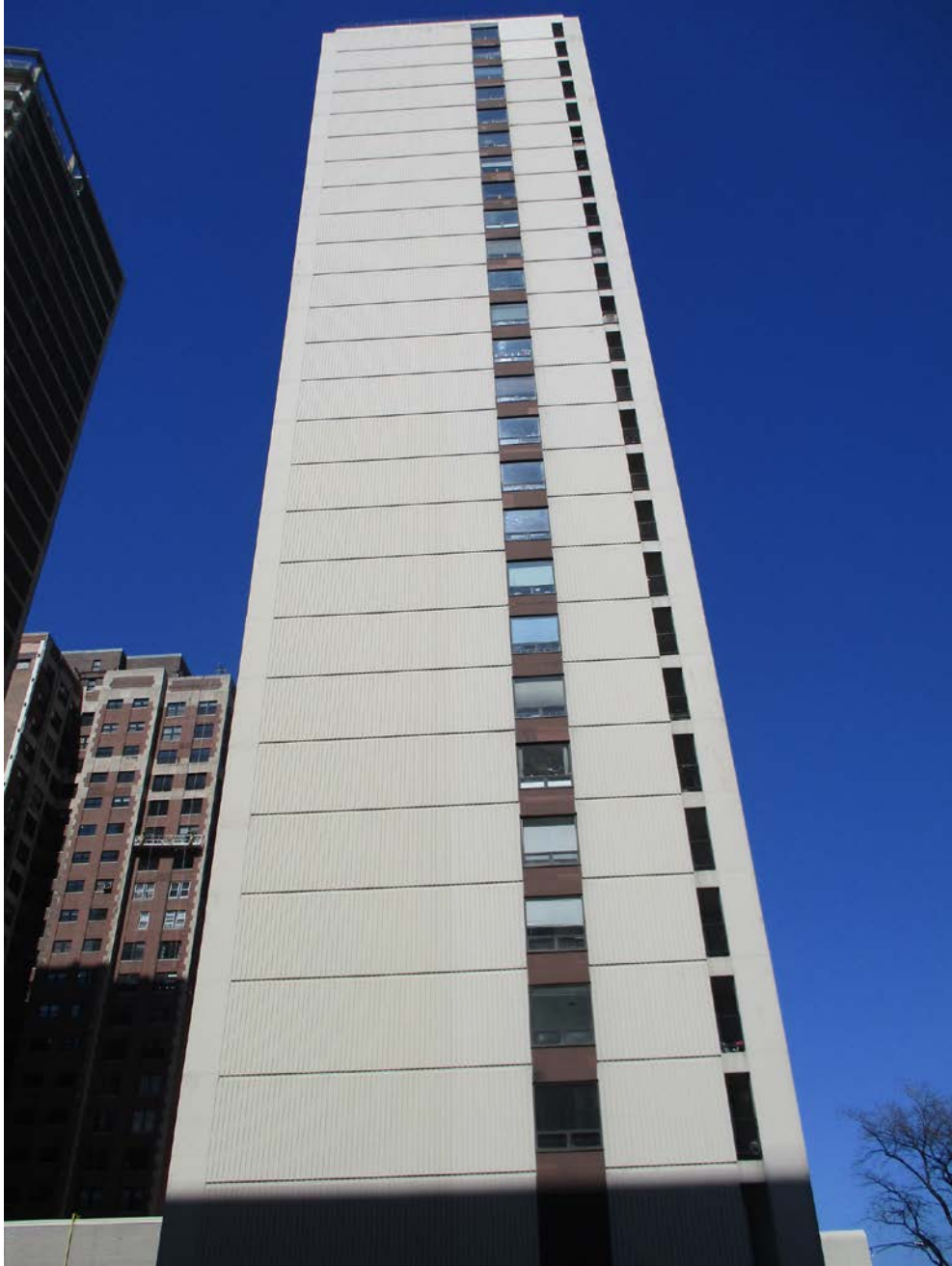
3200 N. Lake Shore Drive, view looking north from W. Belmont Avenue toward South façade
