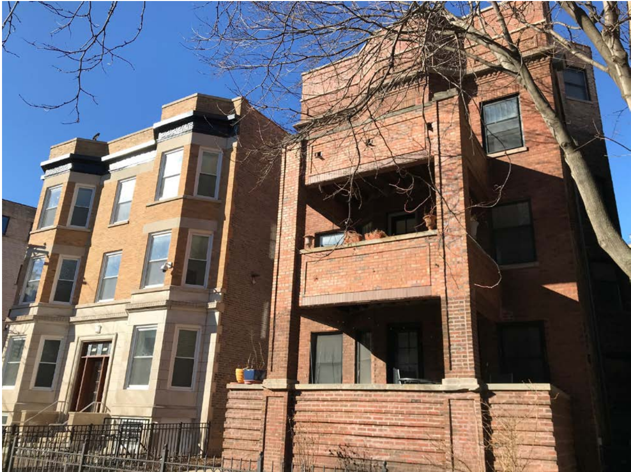
650 W. Grace Street, view looking northwest from W. Grace Street toward South façade
