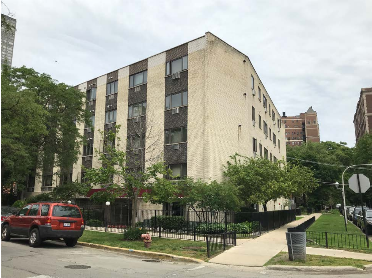
3801 N. Pine Grove Avenue, view looking northeast from N. Pine Grove Avenue toward West façade
