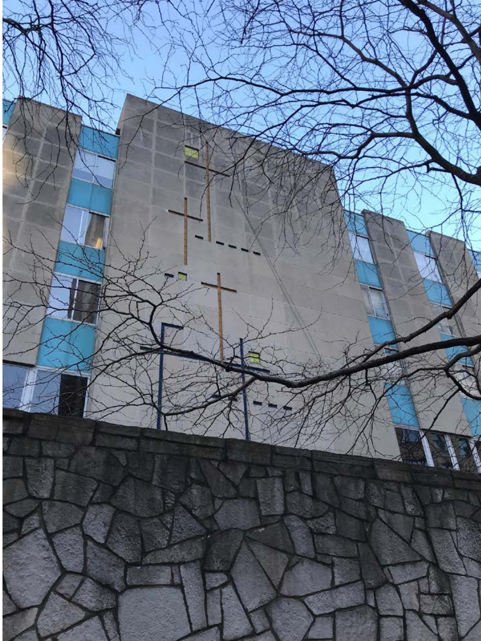
2913 N. Commonwealth Avenue, view looking east from N. Commonwealth Avenue toward West façade detailing
