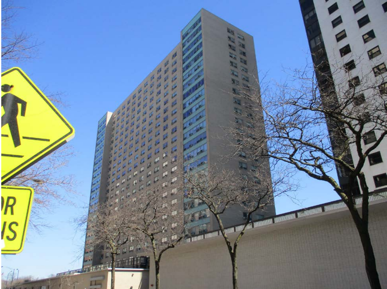
3180 N. Lake Shore Drive, view looking northeast from N. Sheridan Road toward West and South façades
