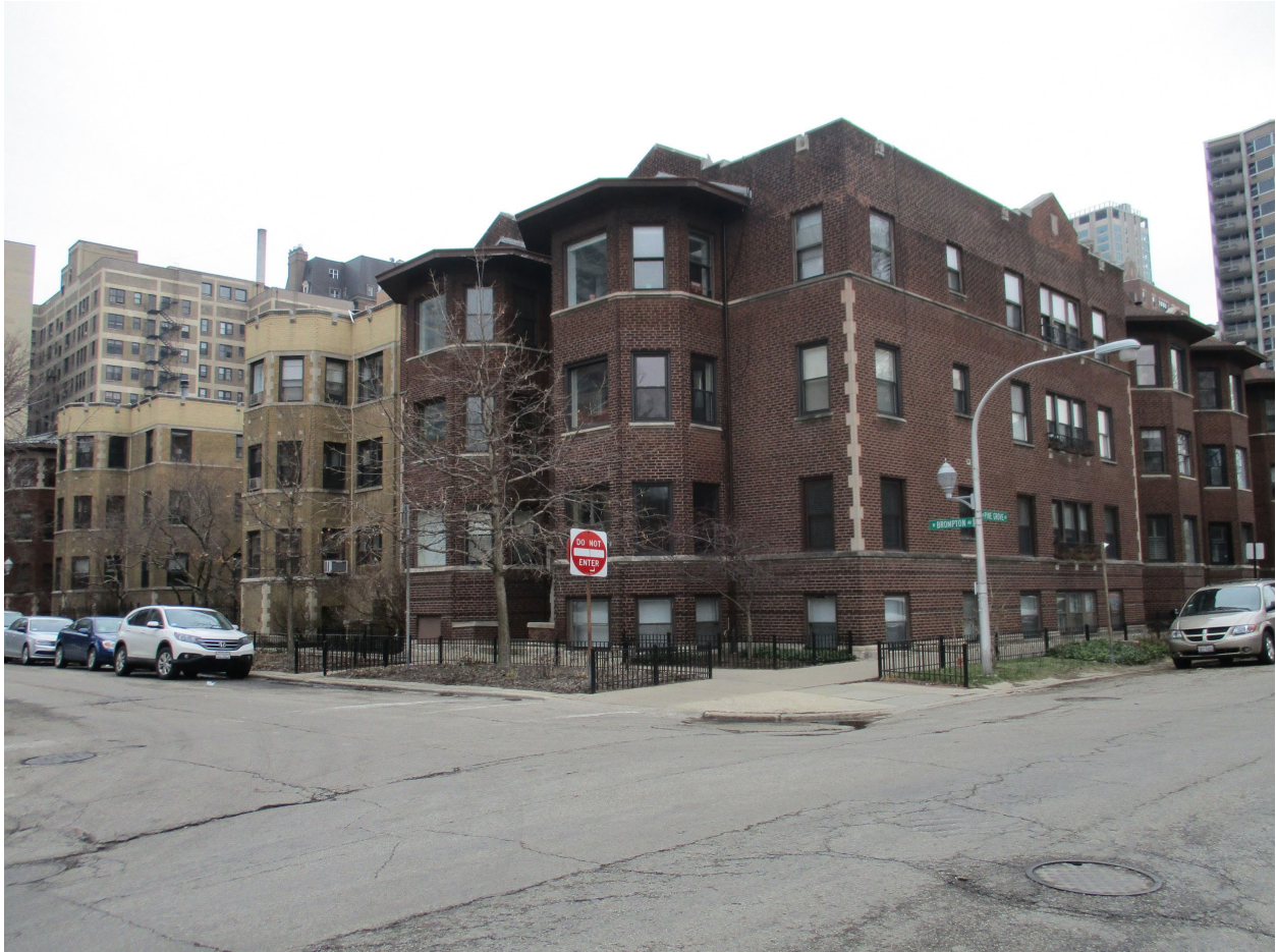
3511-3519 N. Pine Grove Avenue/ 549-551 W. Brompton Avenue, view looking southeast from the intersection of N. Pine Grove Avenue and W. Brompton Avenue toward North and West façades
