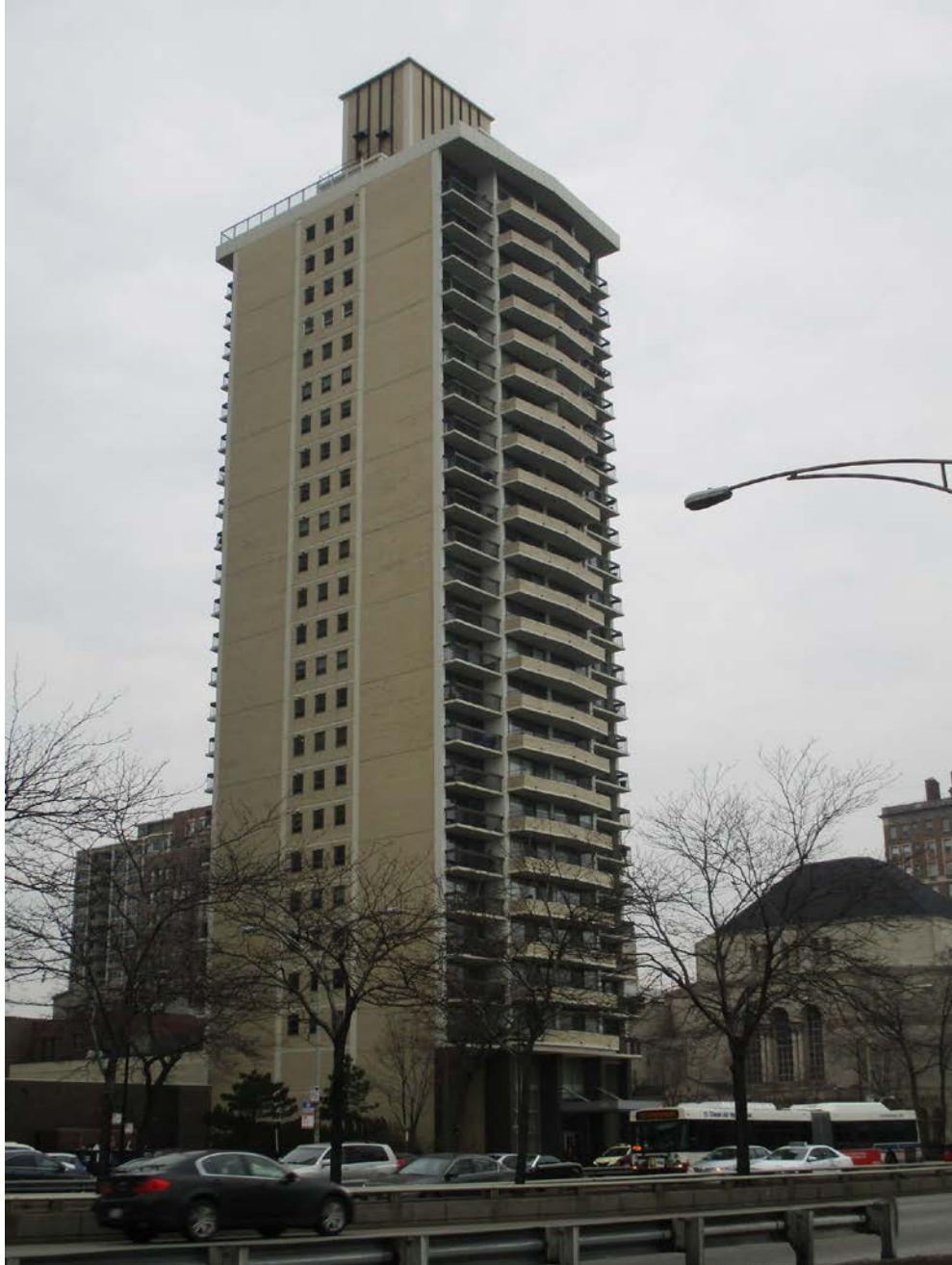
3470 N. Lake Shore Drive, view looking northwest from N. Lake Shore Drive toward South and East façades
