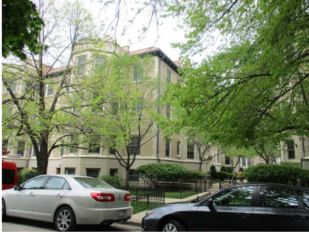
534-552 W. Brompton Avenue, view looking northwest from W. Brompton Avenue toward South façade of middle mass
