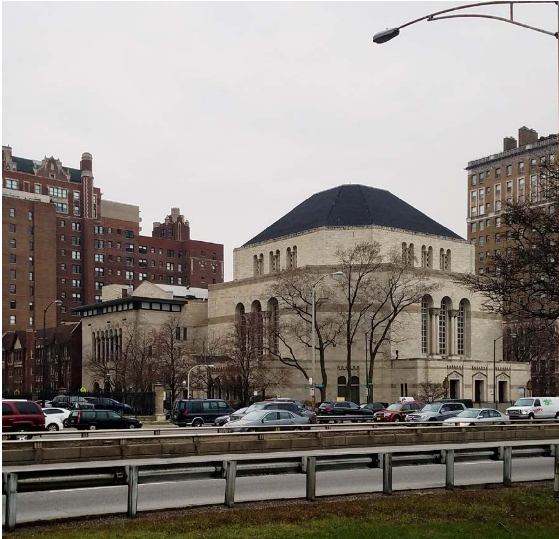
3480 N. Lake Shore Drive/ 513 W. Cornelia Avenue, view looking northwest from N. Lake Shore Drive toward South and East façades
