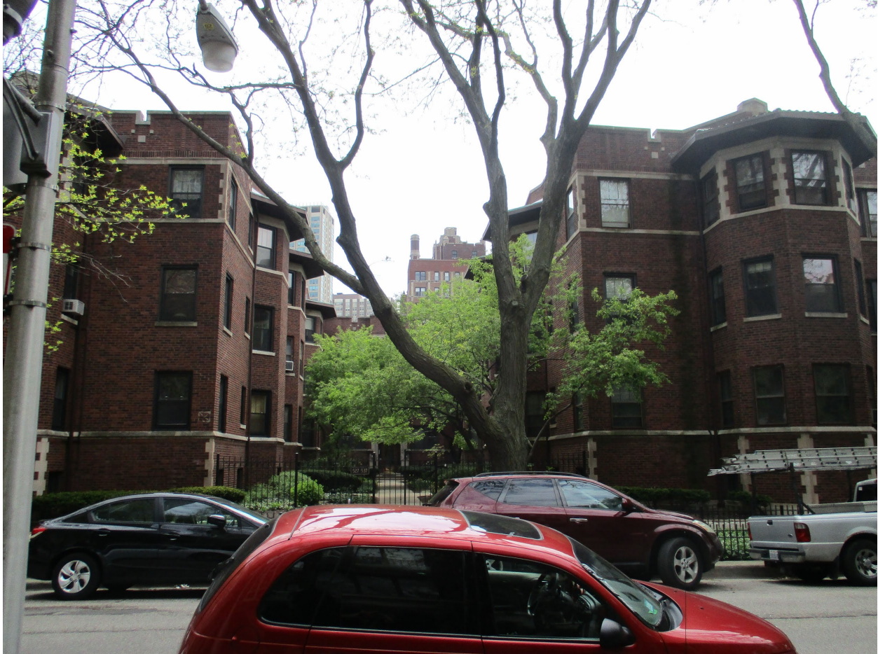
527-537 W. Brompton Avenue, view looking south from W. Brompton Avenue toward courtyard
