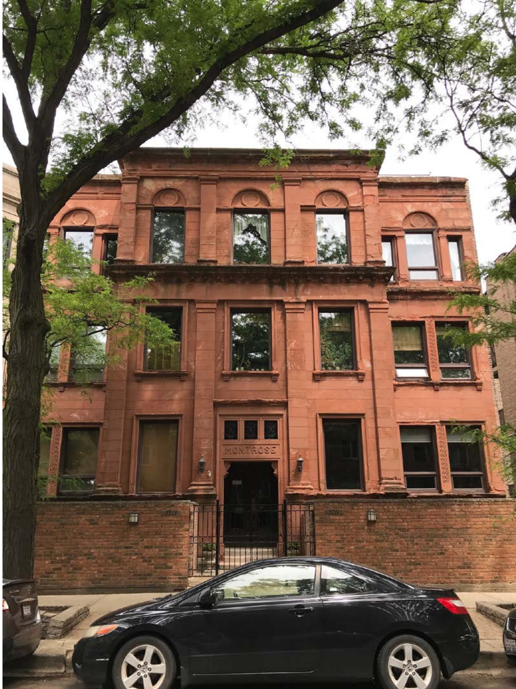
3711-3713 N. Pine Grove Avenue, view looking east from N. Pine Grove Avenue toward West façade
