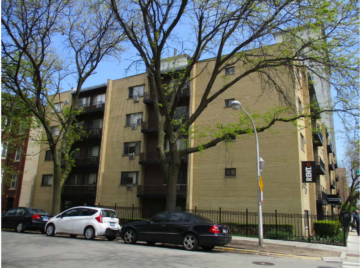
536 W. Addison Street, view looking northeast from N. Pine Grove Avenue toward West façade
