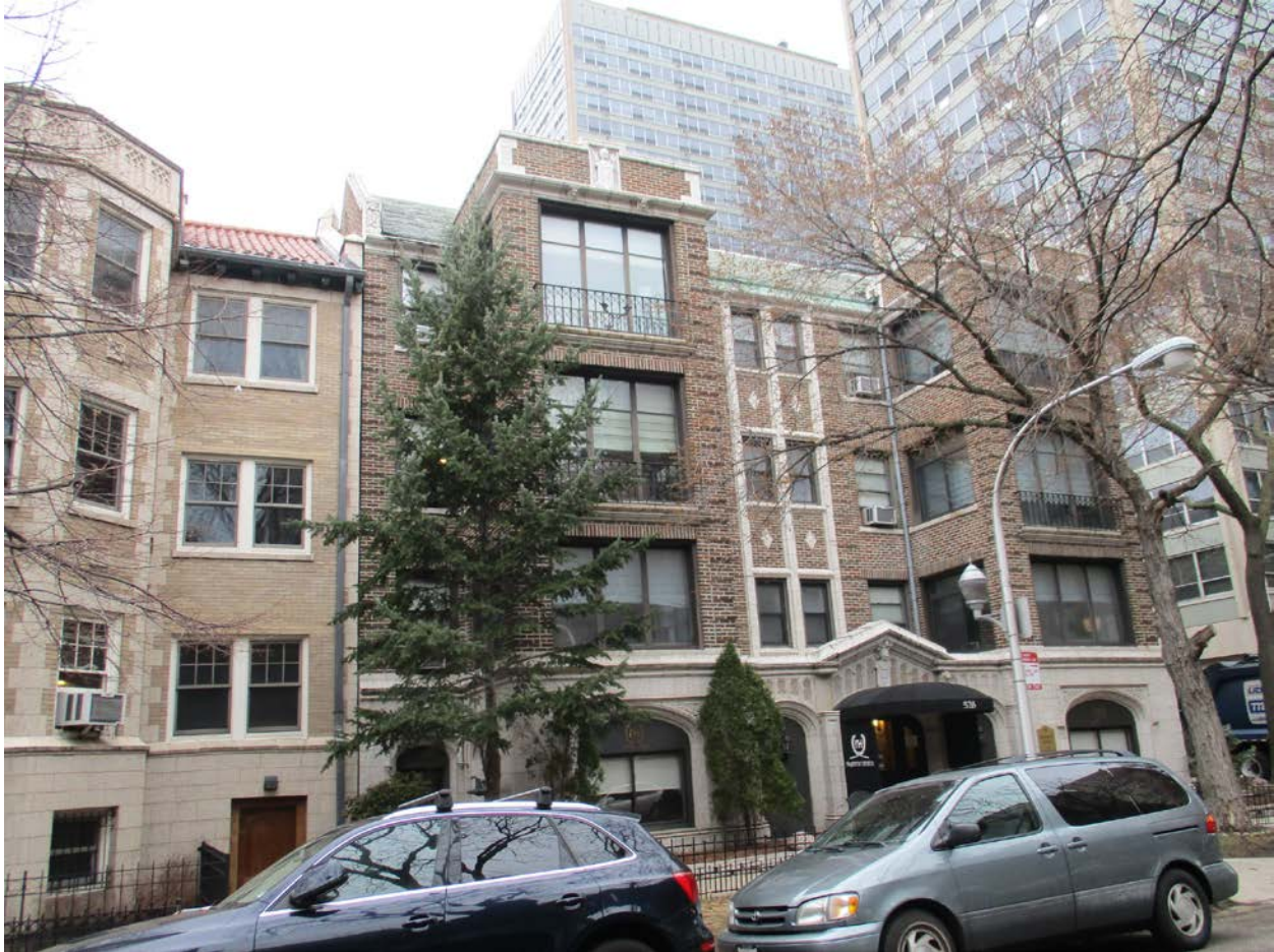
528 W. Brompton Avenue, view looking northeast from W. Brompton Avenue toward South façade
