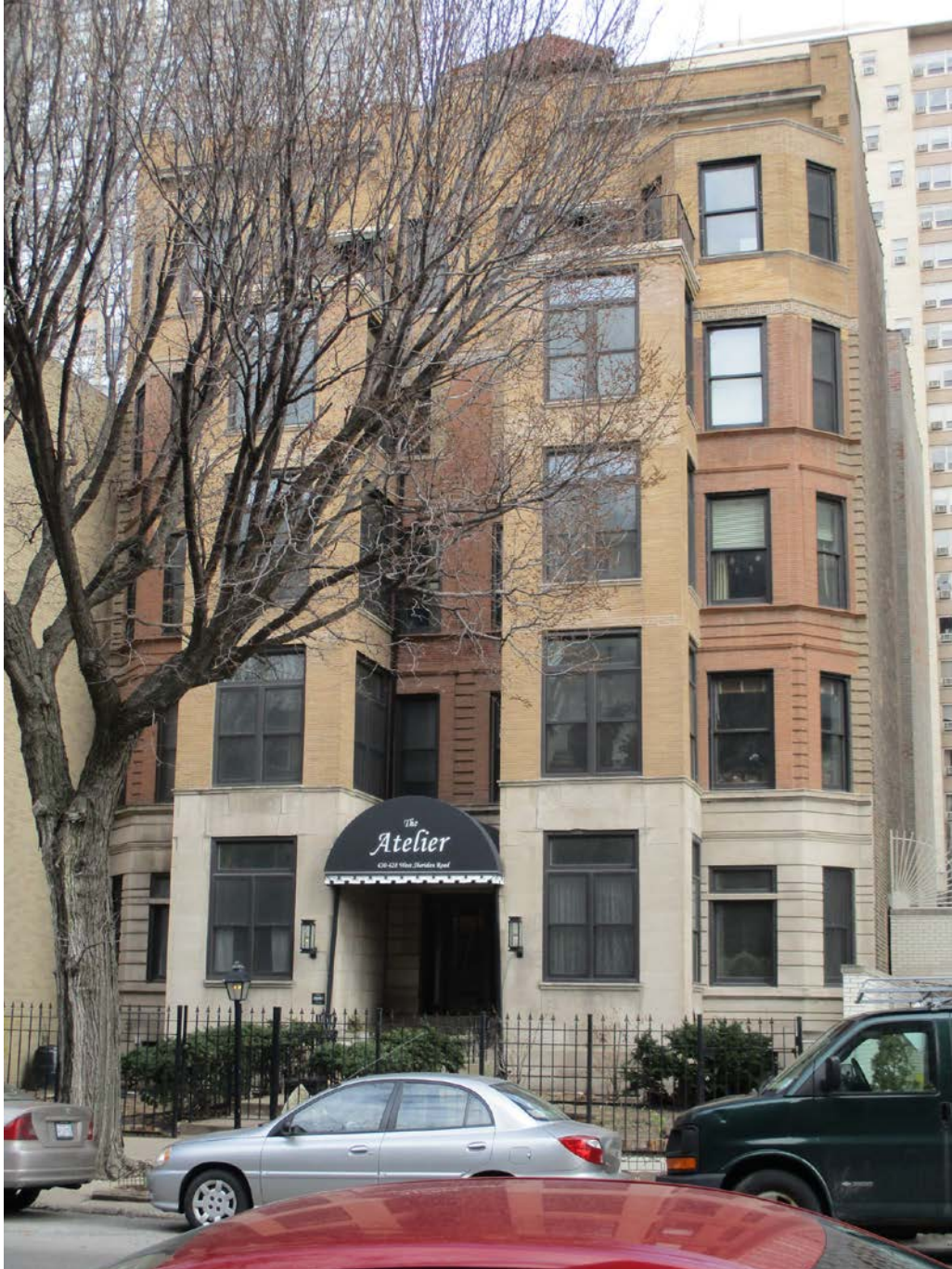
628-630 W. Sheridan Road, view looking north from W. Sheridan Road toward South façade
