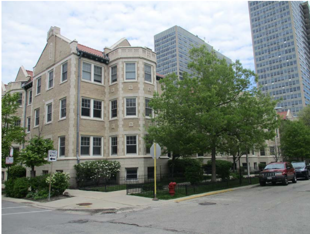
534-552 W. Brompton Avenue, view looking northeast from intersection of W. Brompton Avenue and N. Pine Grove Avenue toward West and South façades of West mass
