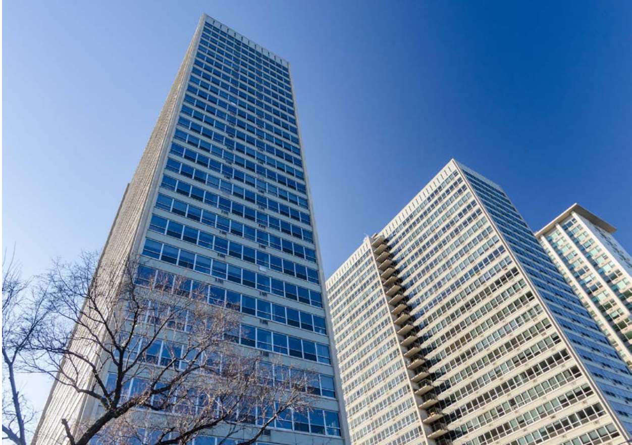
3550 N. Lake Shore Drive, view looking northwest from N. Lake Shore Drive toward the East façade of the South Tower and the South façade of the North Tower
