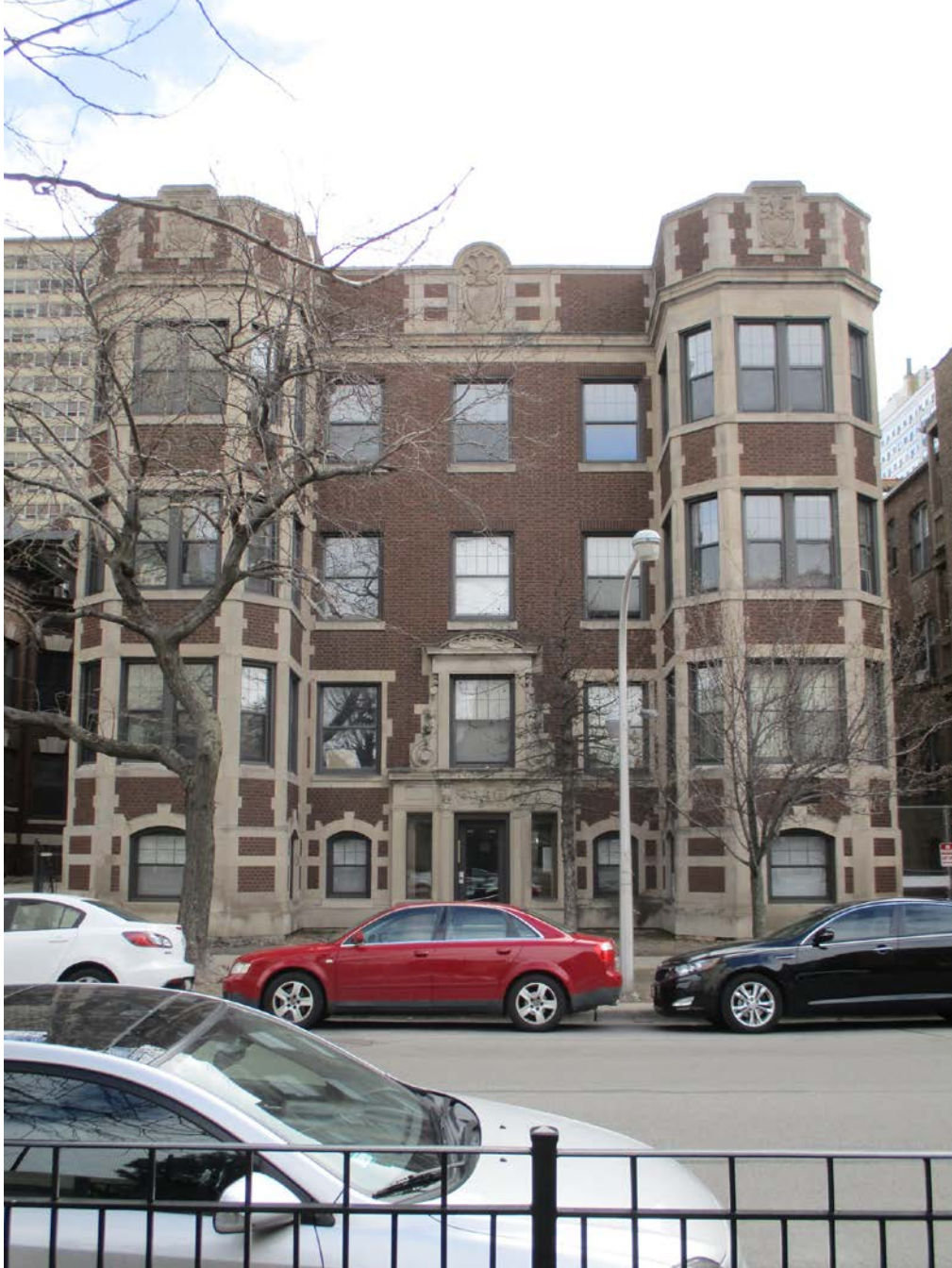
3933-3935 N. Pine Grove Avenue, view looking east from N. Pine Grove Avenue toward West façade
