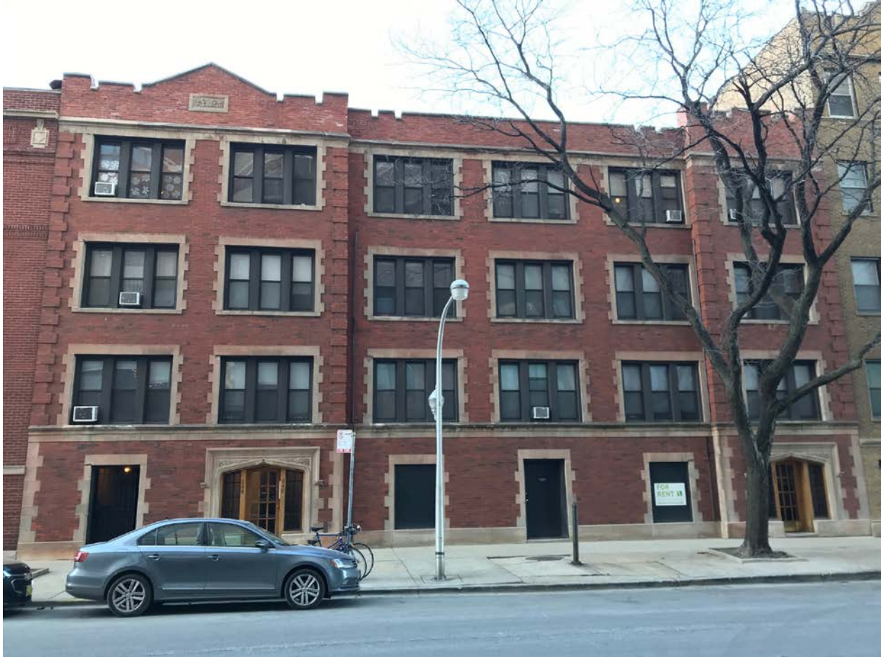
642-648 W. Waveland Avenue, view looking north from W. Waveland Avenue toward South façade
