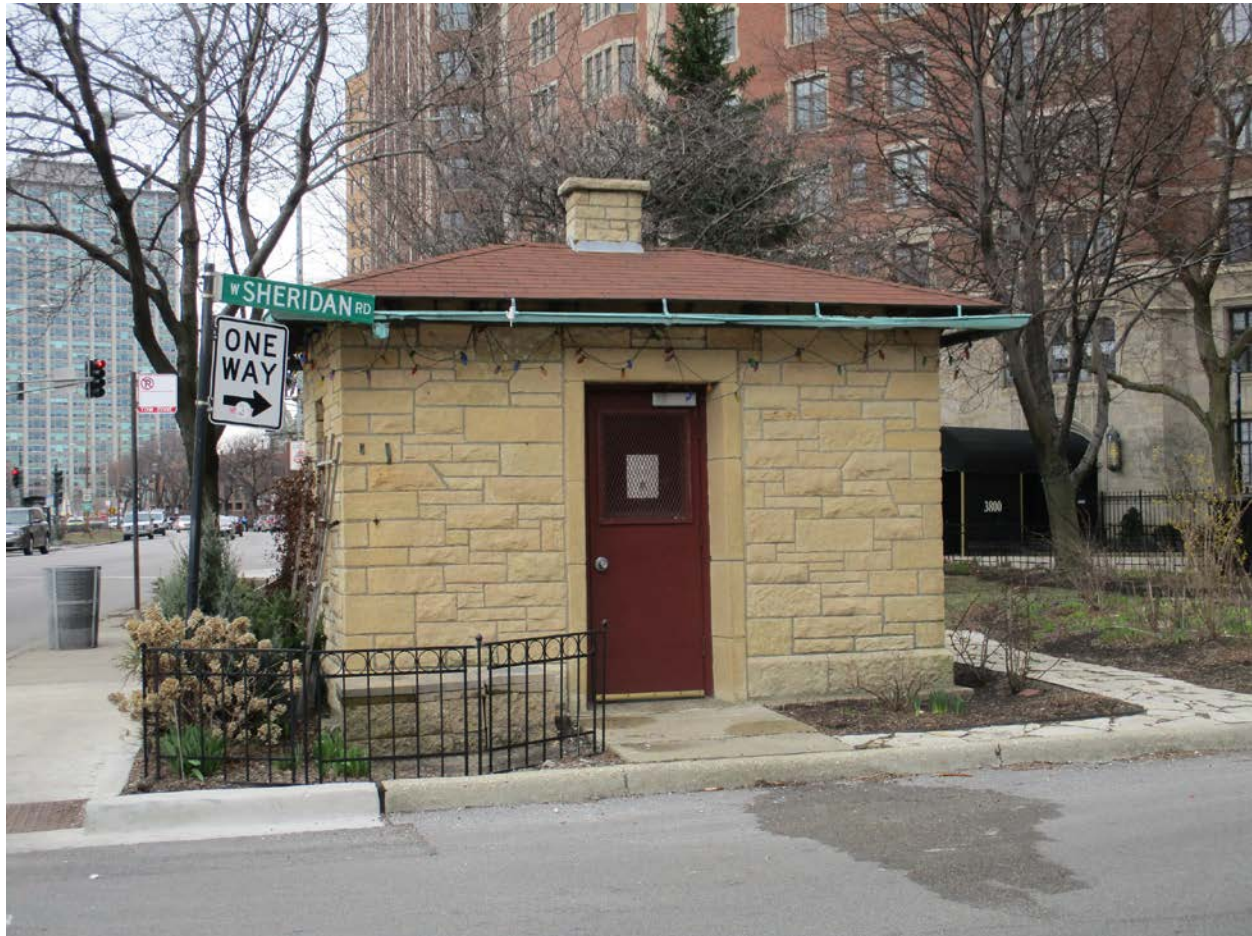
Park Structure, view looking southwest from W. Sheridan Road toward North façade
