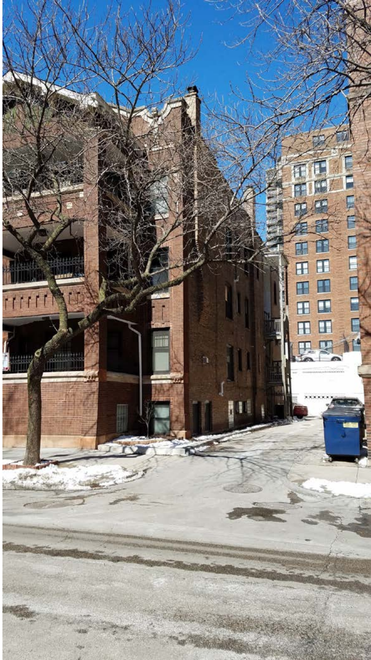
416 W. Briar Place, view looking northwest from W. Briar Place toward East façade
