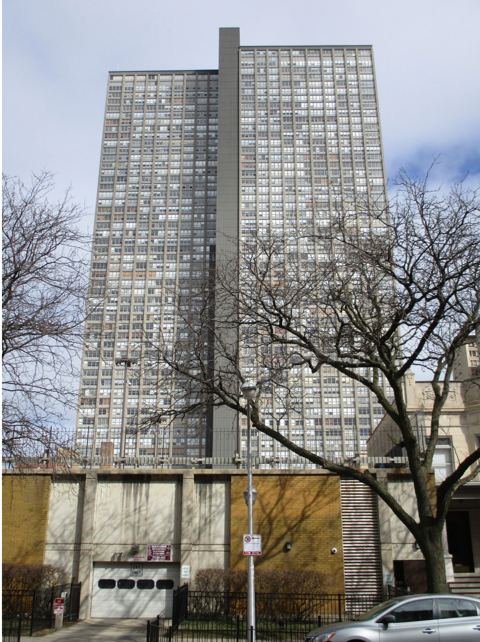
655 W. Irving Park Road, view looking north from W. Sheridan Road toward South façade
