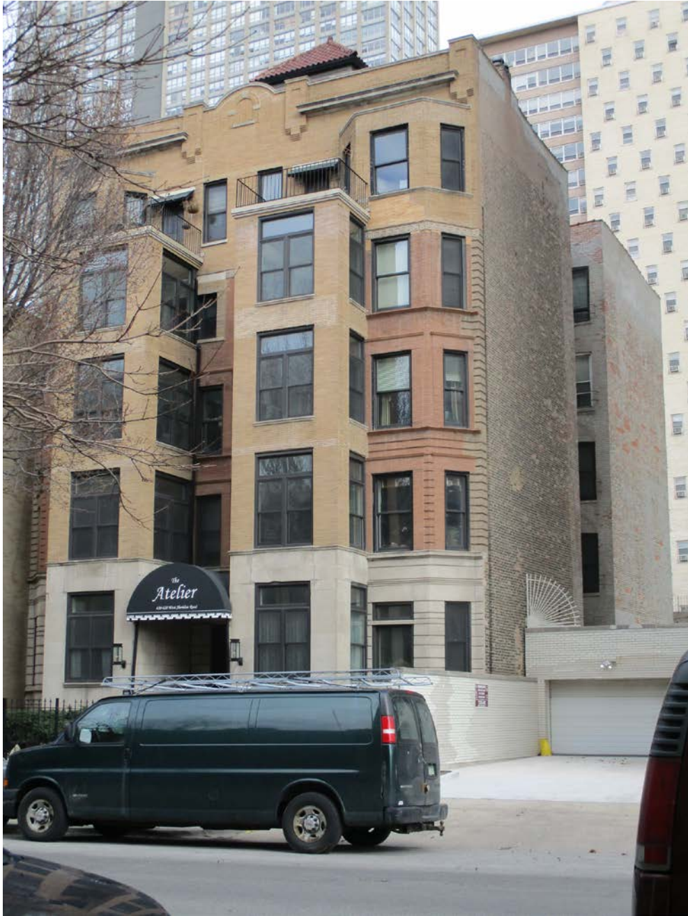
628-630 W. Sheridan Road, view looking northwest from W. Sheridan Road toward South and East façades
