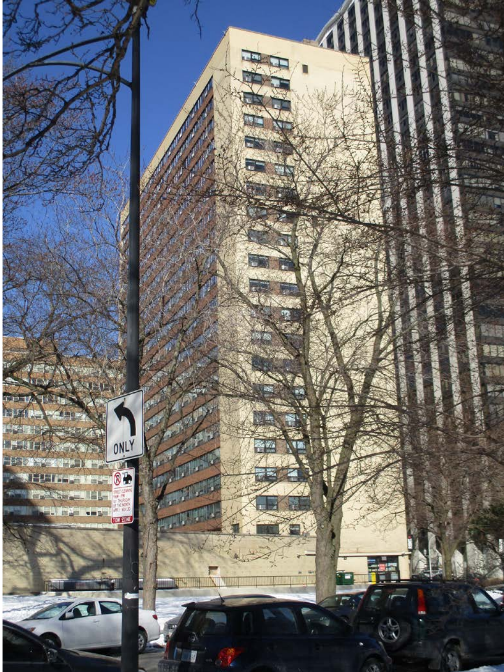
3130 N. Lake Shore Drive, view looking northwest from N. Lake Shore Drive toward East façade
