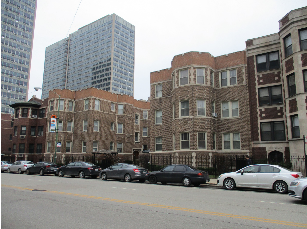
541-549 W. Addison Street, view looking southeast from W. Addison Street toward North façades
