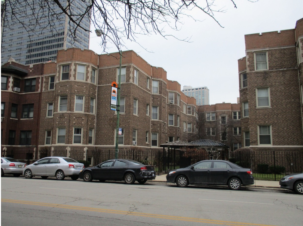
541-549 W. Addison Street, view looking southeast from W. Addison Street toward North and West façades of East mass
