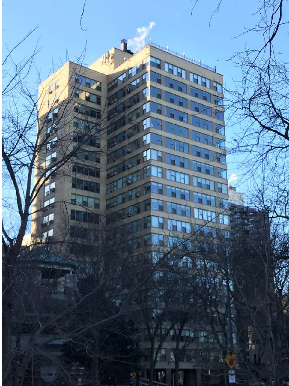
2970 N. Lake Shore Drive, view looking northwest from N. Lake Shore Drive toward South and East façades
