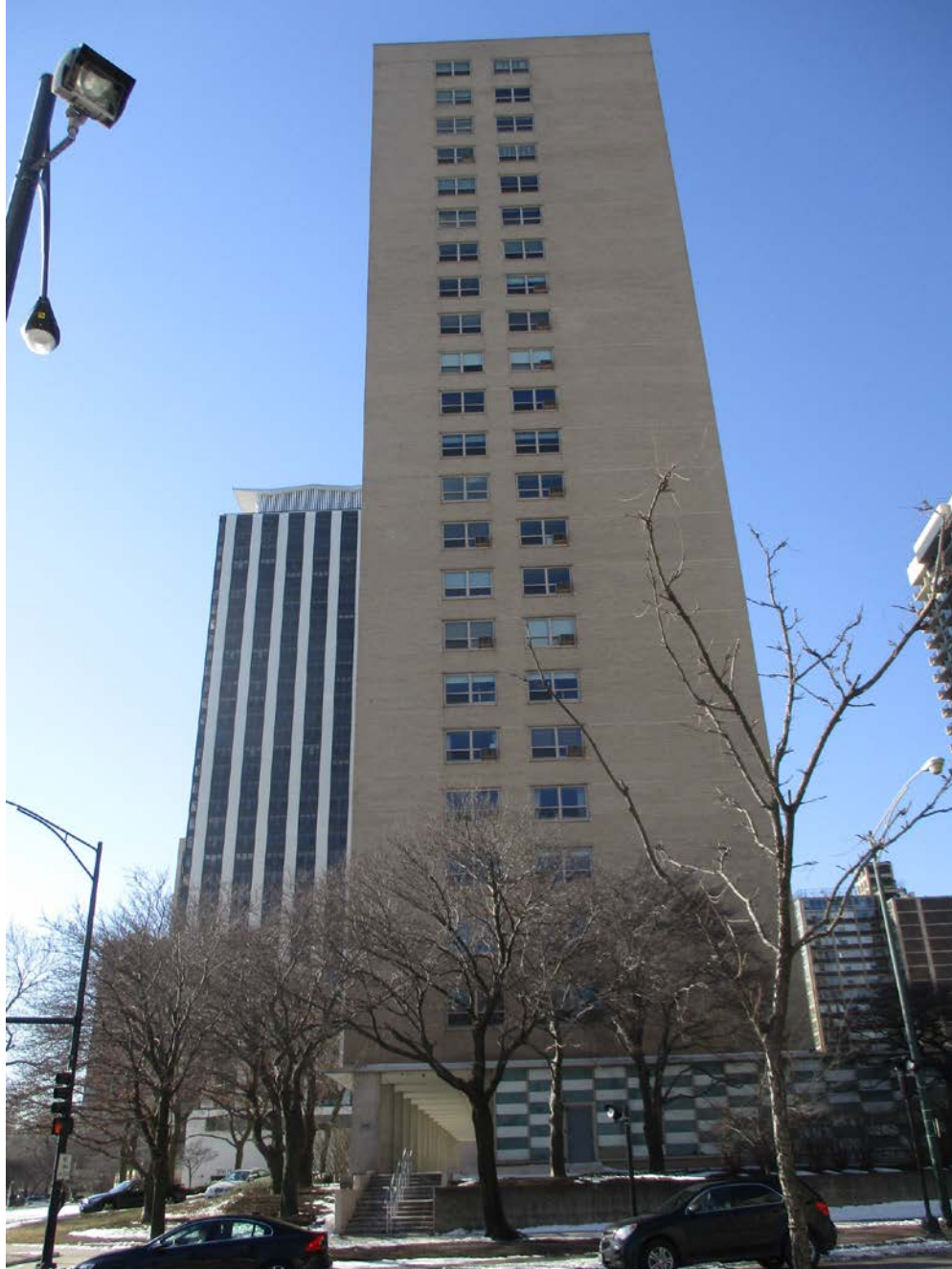
3180 N. Lake Shore Drive, view looking south from W. Belmont Avenue toward North façade
