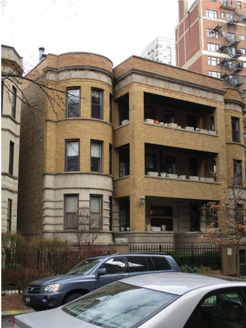
626-628 W. Grace Street, view looking northeast from W. Grace Street toward West and South façades
