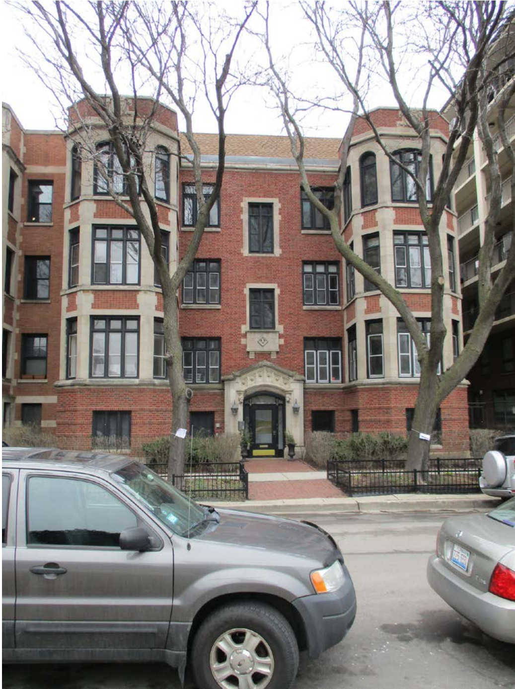
616-618 W. Waveland Avenue, view looking north from W. Waveland Avenue toward South façade
