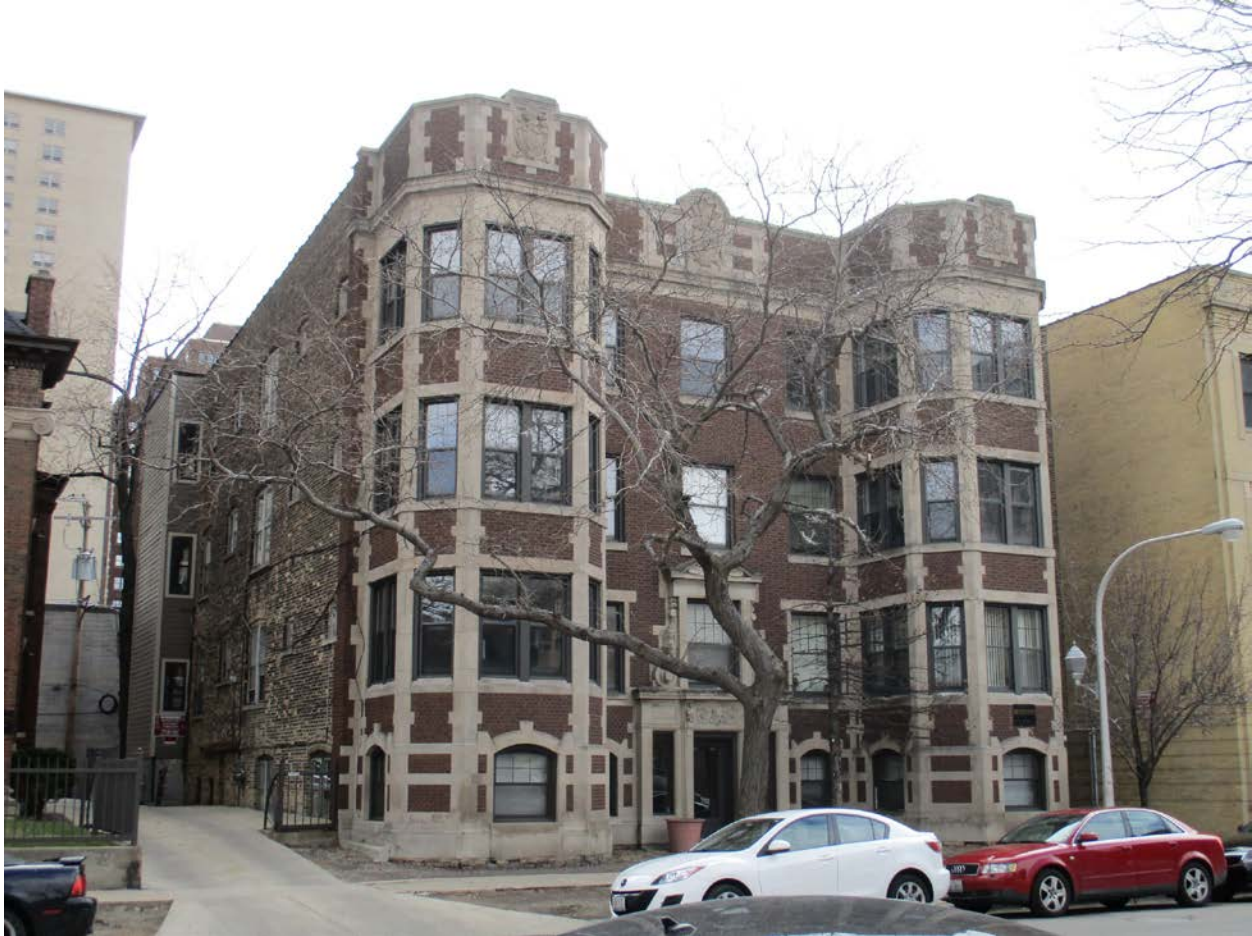
3933-3935 N. Pine Grove Avenue, view looking southeast from N. Pine Grove Avenue toward North and West façade
