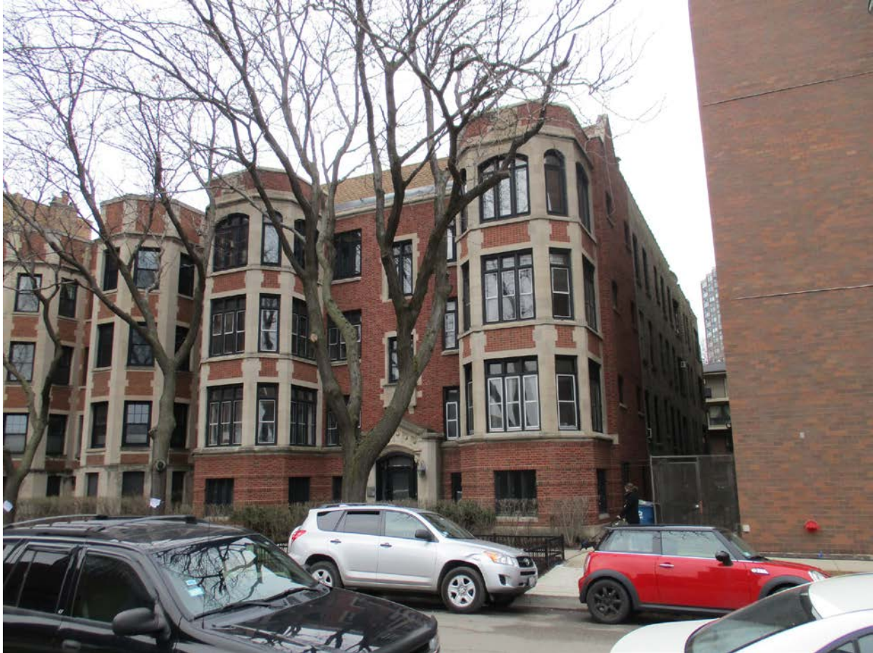
616-618 W. Waveland Avenue, view looking northwest from W. Waveland Avenue toward South and East façades
