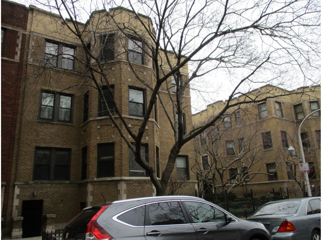
539-547 W. Brompton Avenue, view looking southwest from W. Brompton Avenue toward North façade of East mass
