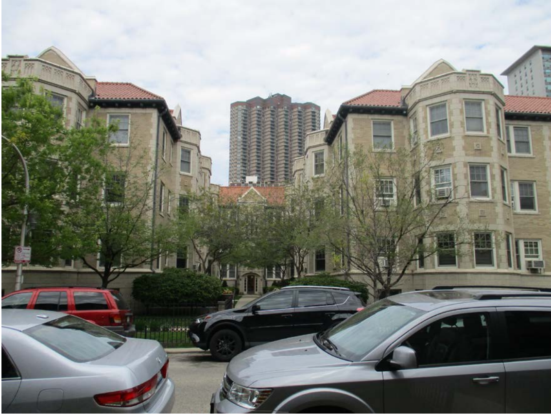
534-552 W. Brompton Avenue, view looking north from W. Brompton Avenue toward West courtyard
