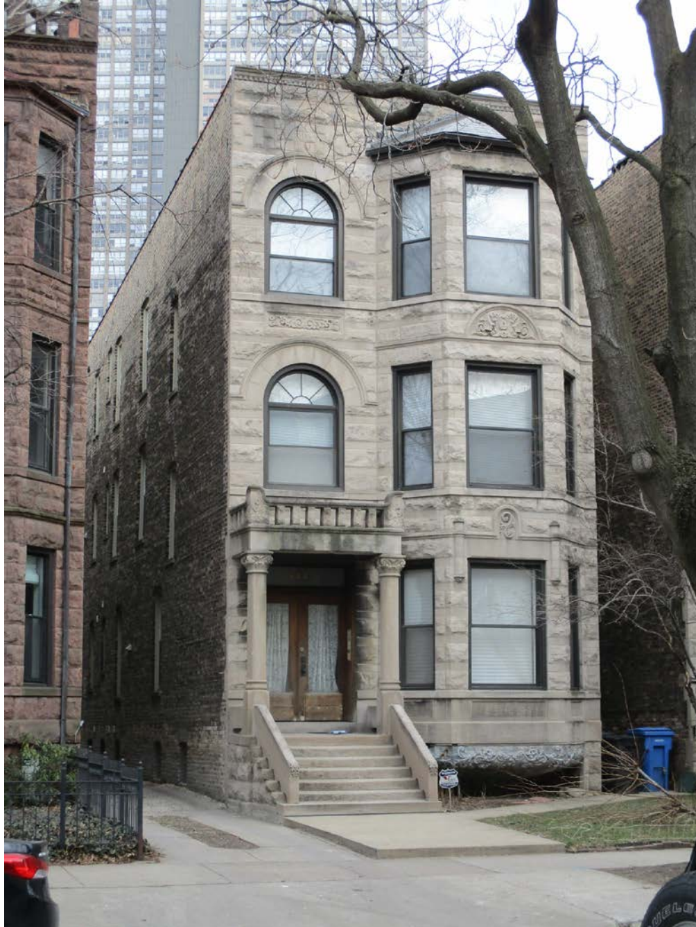
644 W. Grace Street, view looking northeast from W. Grace Street toward West and South façades
