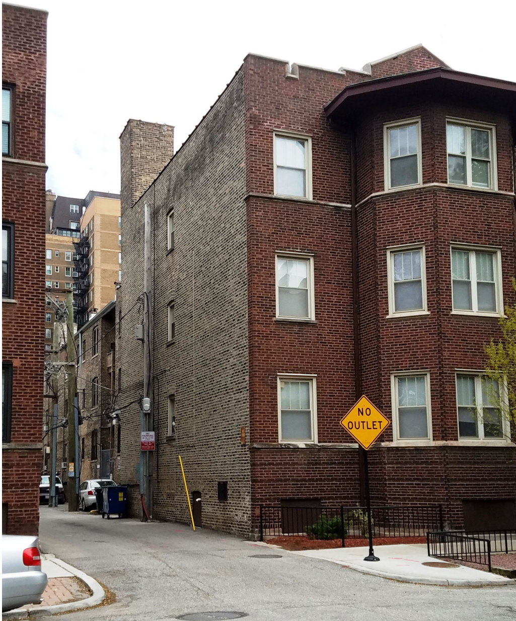
3501-3507 N. Pine Grove Avenue/ 546 W. Cornelia Avenue, view looking southeast from N. Pine Grove Avenue toward North façade
