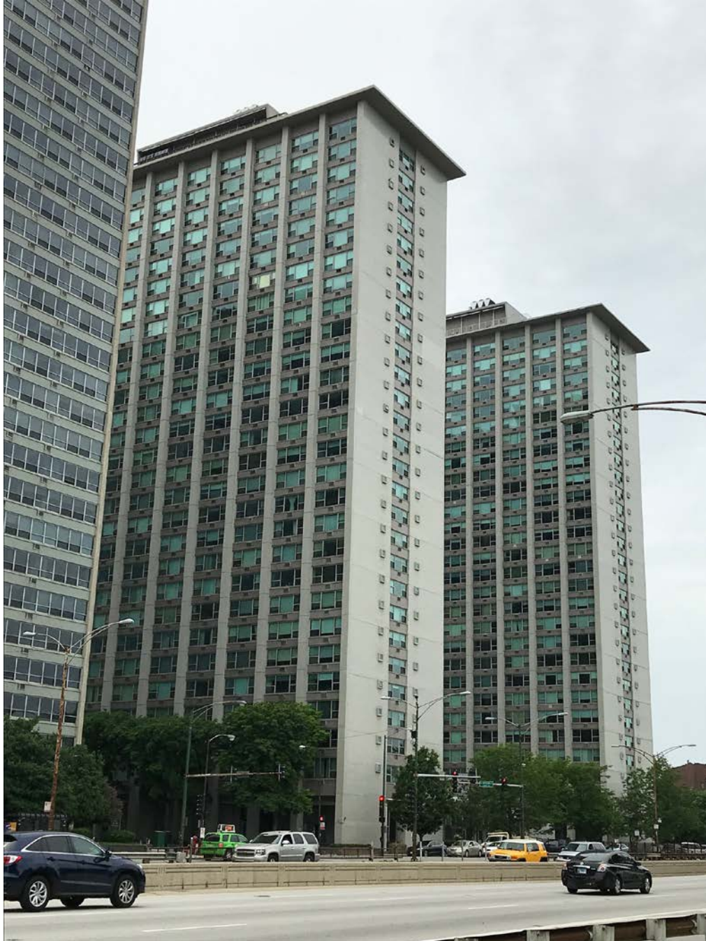
3600 N. Lake Shore Drive, view looking northwest from N. Lake Shore Drive toward South and East façades
