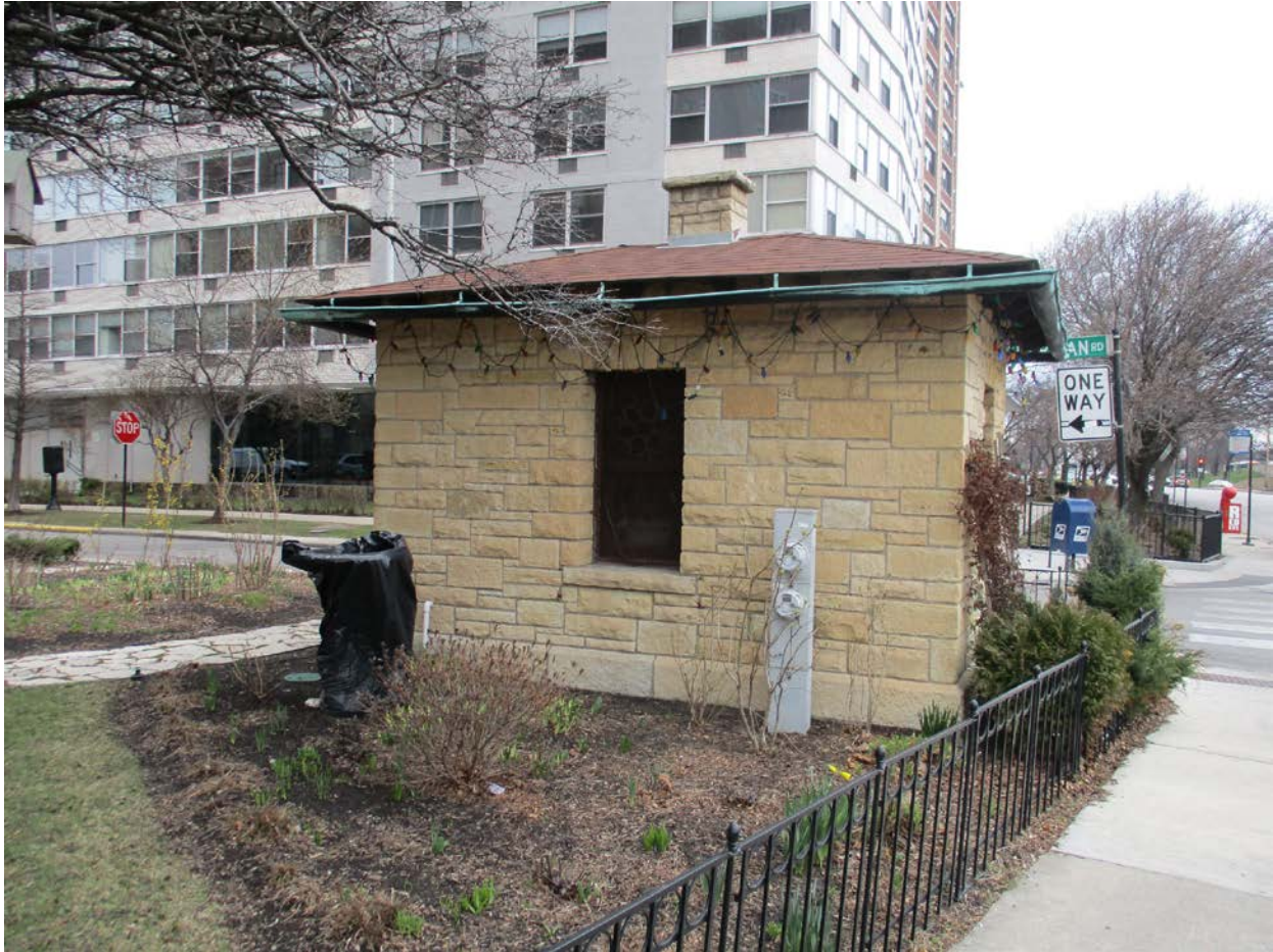
Park Structure, view looking northwest from N. Lake Shore Drive toward South façade
