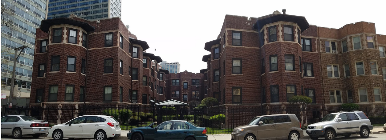
531-539 W. Addison Street, view looking south from W. Addison Street toward courtyard and North façades
