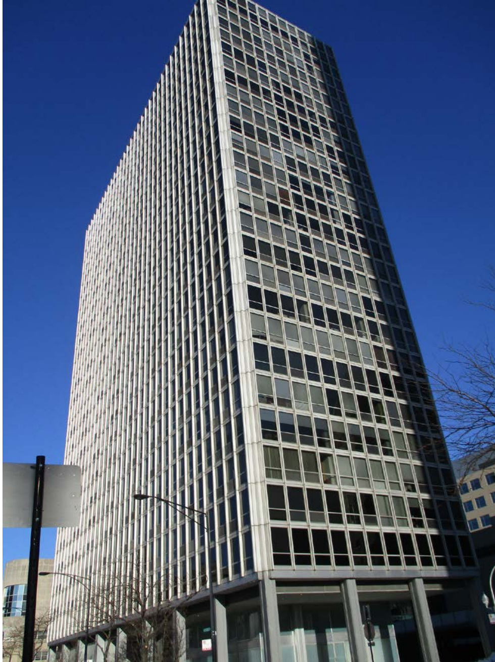
330-340 W. Diversey Parkway, view looking northwest from W. Diversey Parkway toward South and East façades of South Tower (330)
