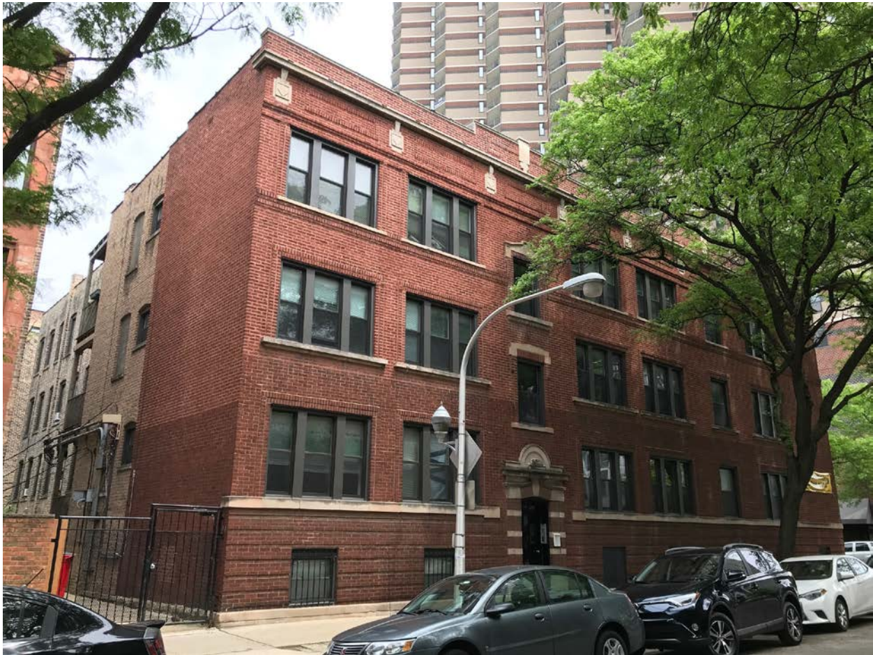
3707-3709 N. Pine Grove Avenue/ 650-652 W. Waveland Avenue, view looking southeast from N. Pine Grove Avenue toward North and West façades
