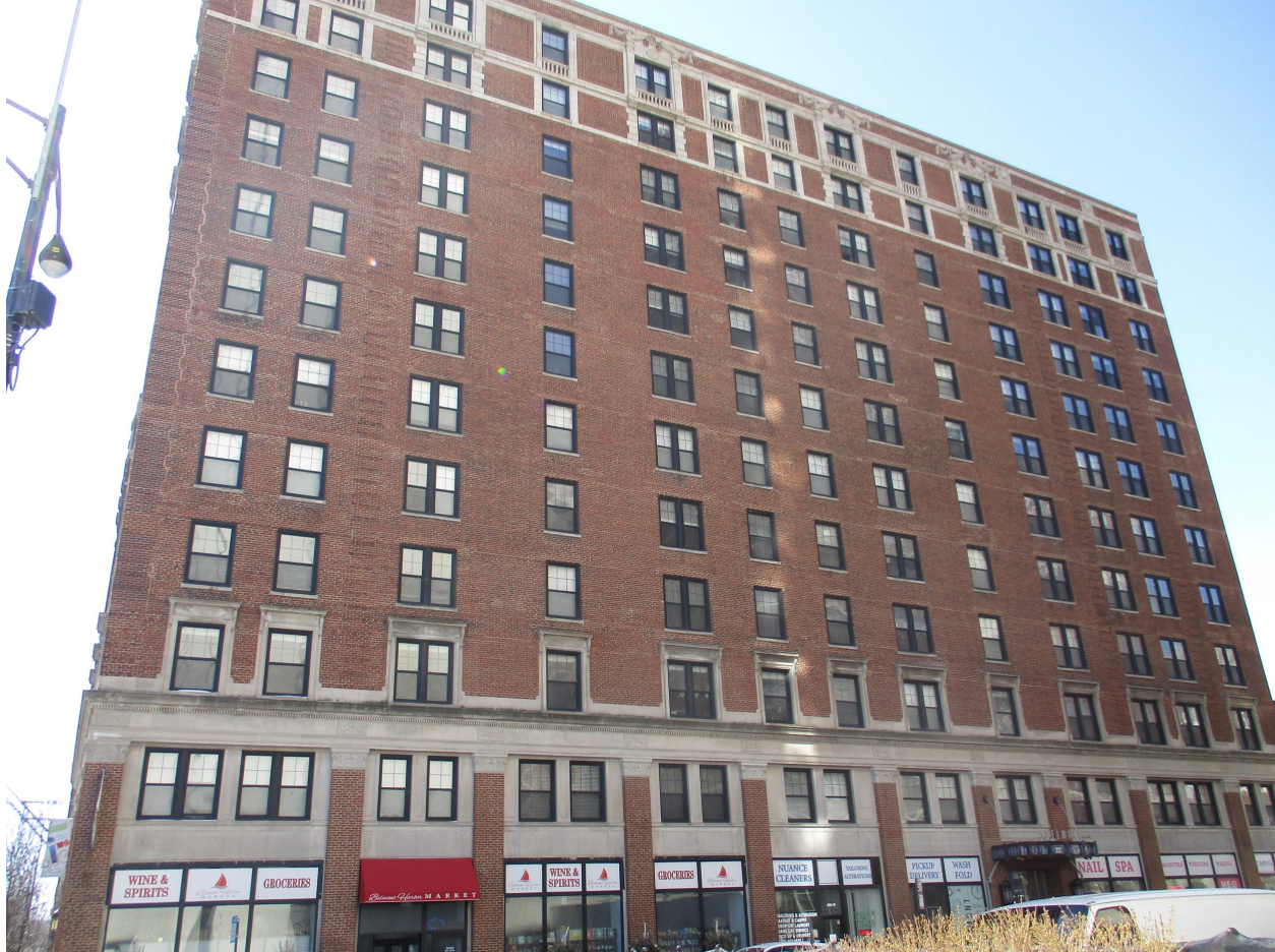
3170 N. Sheridan Road, view looking southwest from W. Belmont Avenue toward North façade
