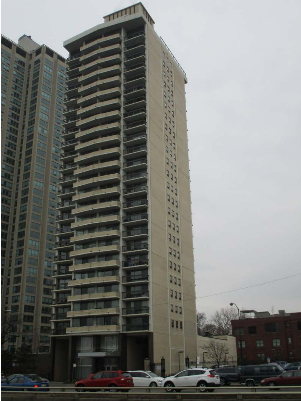
3470 N. Lake Shore Drive, view looking southwest from N. Lake Shore Drive toward East and North façades
