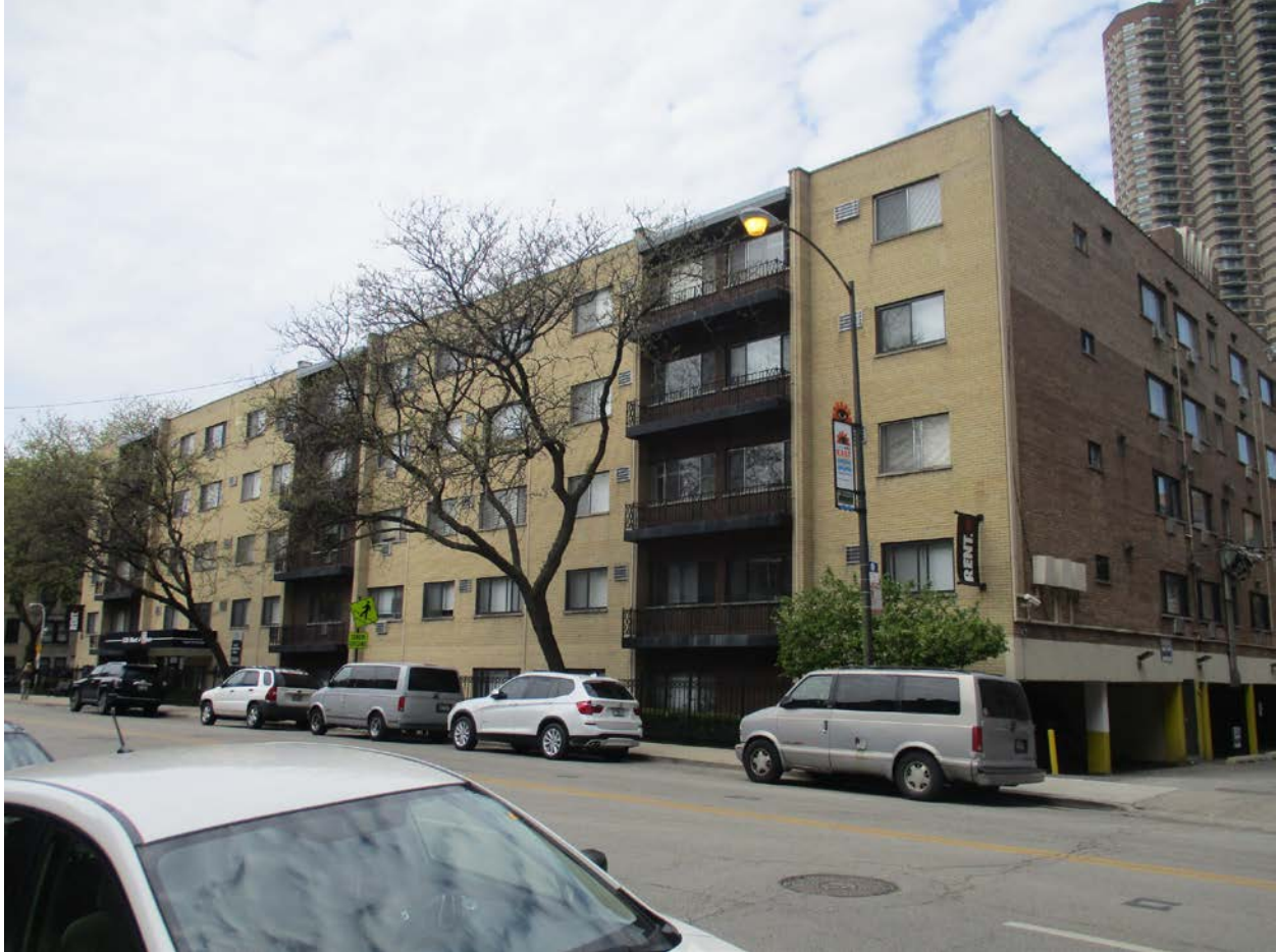
536 W. Addison Street, view looking northwest from W. Addison Street toward East and South façades
