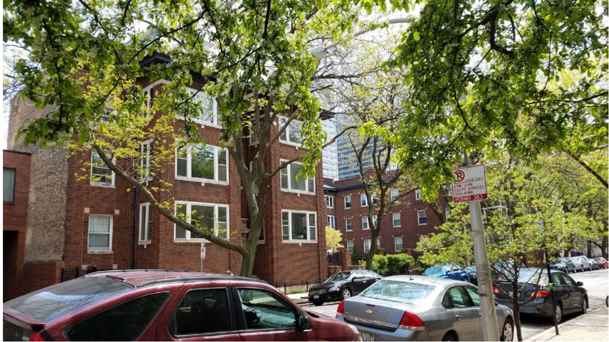
3611-3629 N. Pine Grove Avenue, view looking southeast from N. Pine Grove Avenue toward West façade of North mass
