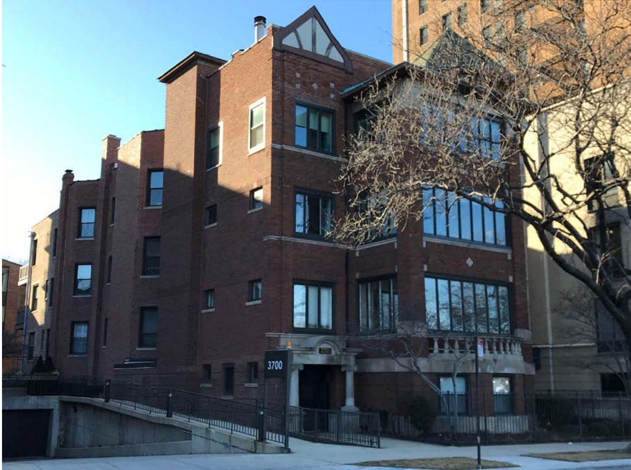
3720 N. Lake Shore Drive, view looking northwest from N. Lake Shore Drive toward East façade
