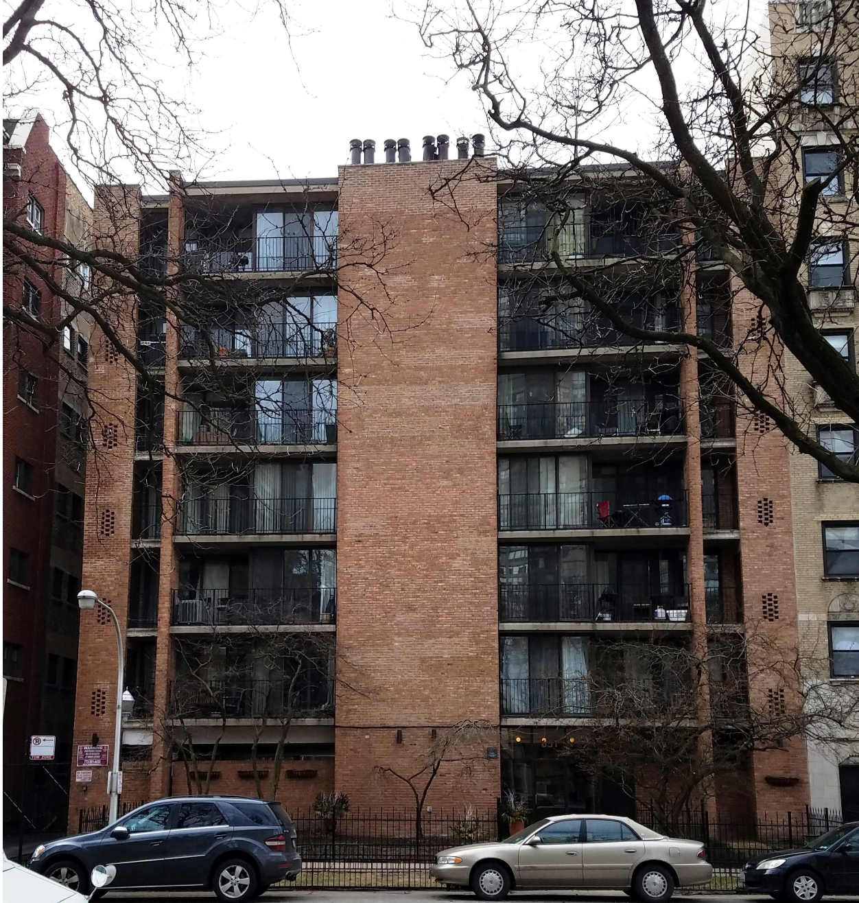
651 W. Sheridan Road, view looking south from W. Sheridan Road toward North façade
