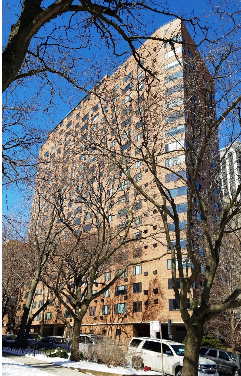
3100 N. Lake Shore Drive/ 316 W. Barry Avenue, view looking northwest from the intersection of N. Lake Shore Drive and W. Barry Avenue toward South façade
