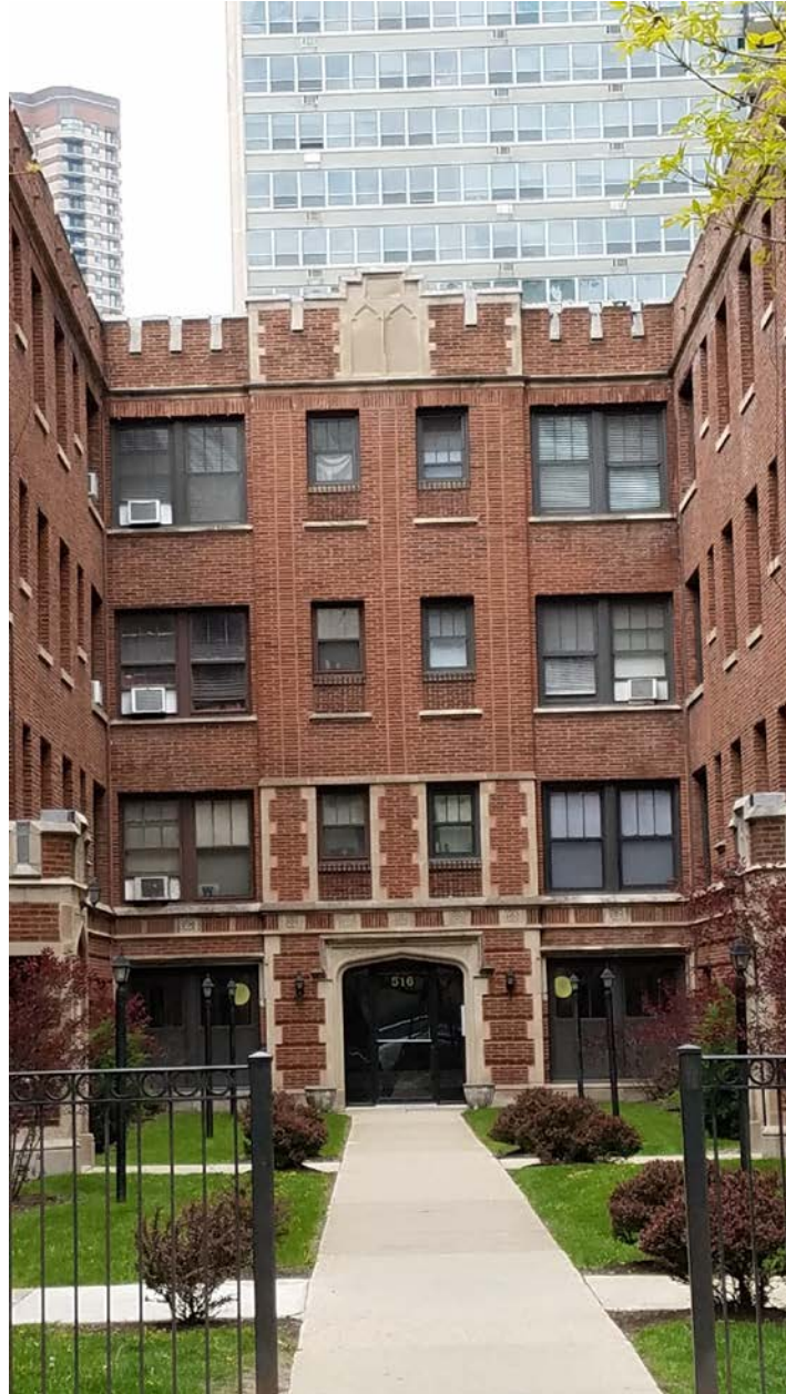
512-520 W. Cornelia Avenue, view looking north from W. Cornelia Avenue toward courtyard
