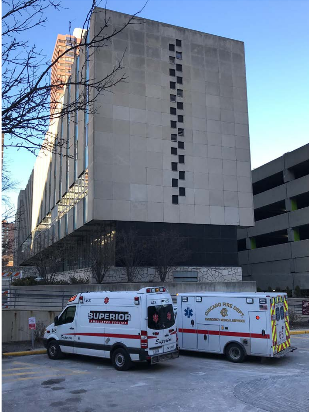
2913 N. Commonwealth Avenue, view looking northeast from N. Commonwealth Avenue toward South façade
