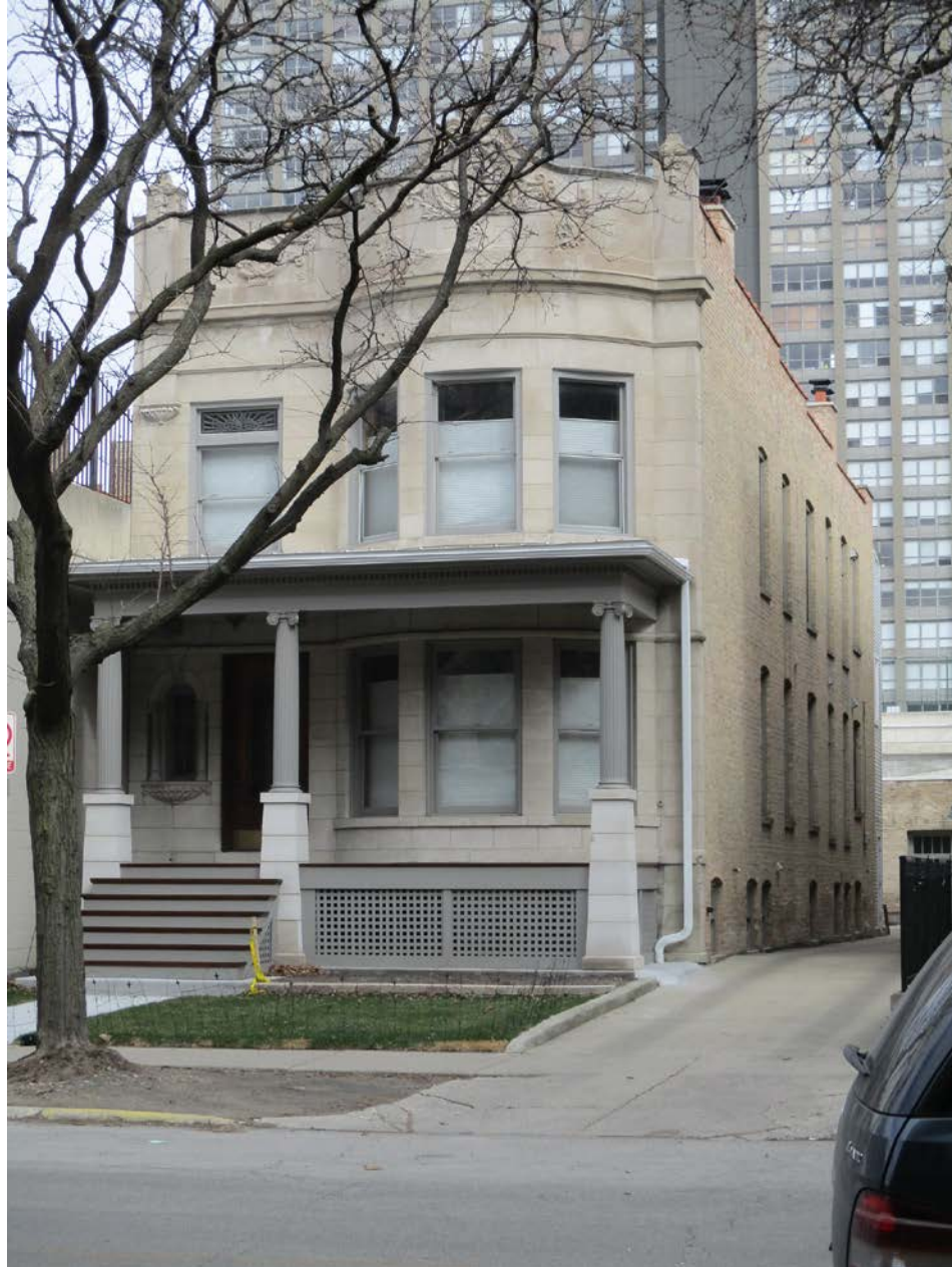
656 W. Sheridan Road, view looking northwest from W. Sheridan Road toward South and East façades
