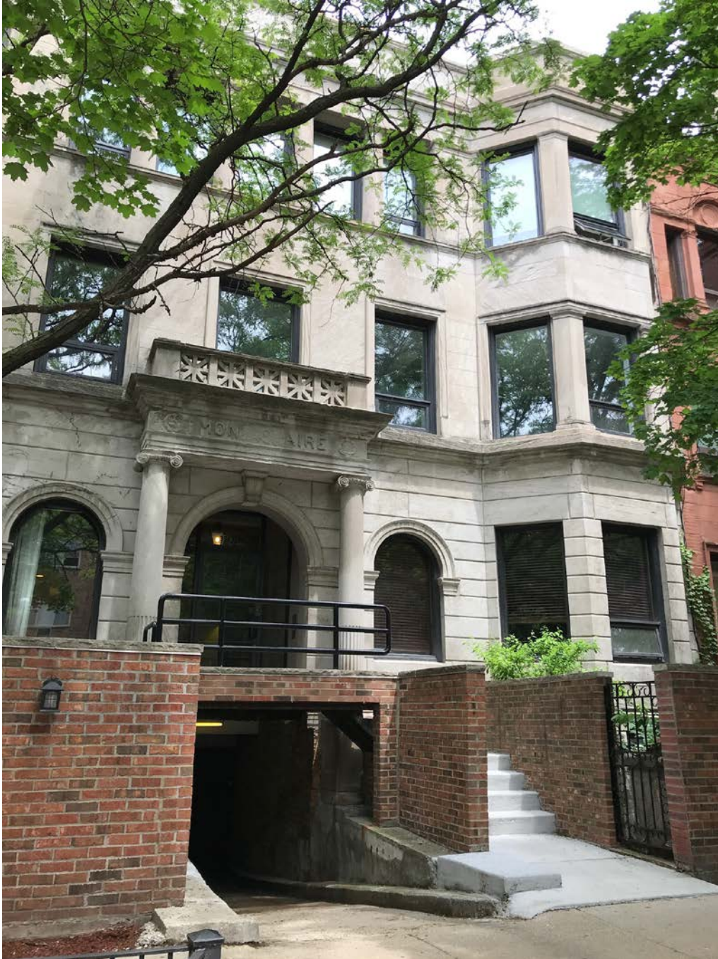
3717-3719 N. Pine Grove Avenue, view looking southeast from N. Pine Grove Avenue toward West façade
