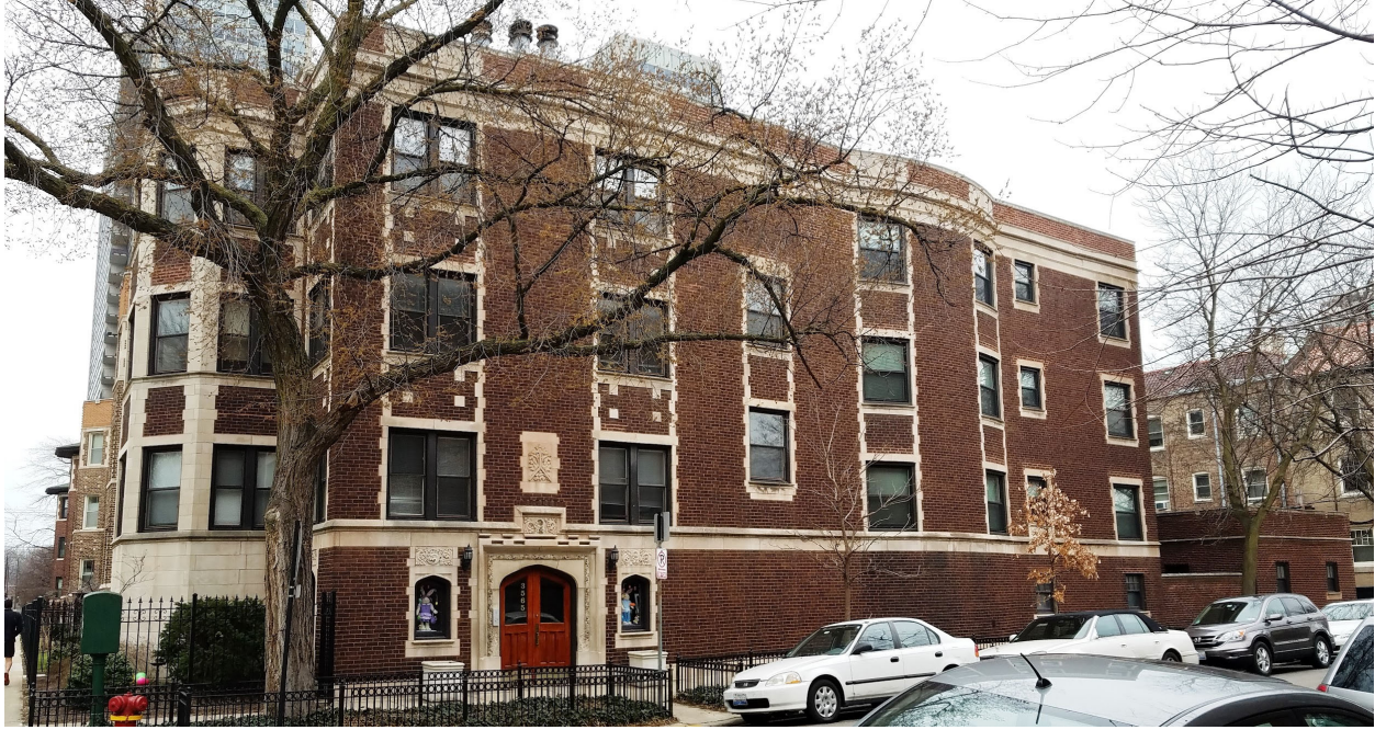
3565 N. Pine Grove Avenue, view looking southeast from N. Pine Grove Avenue toward West façade
