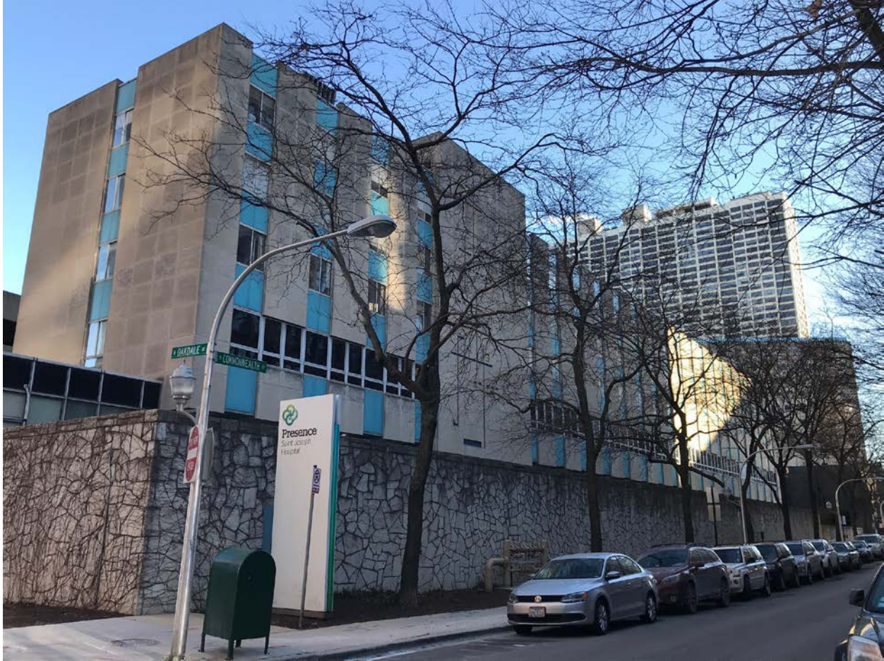
2913 N. Commonwealth Avenue, view looking southeast from W. Oakdale Avenue toward West façade
