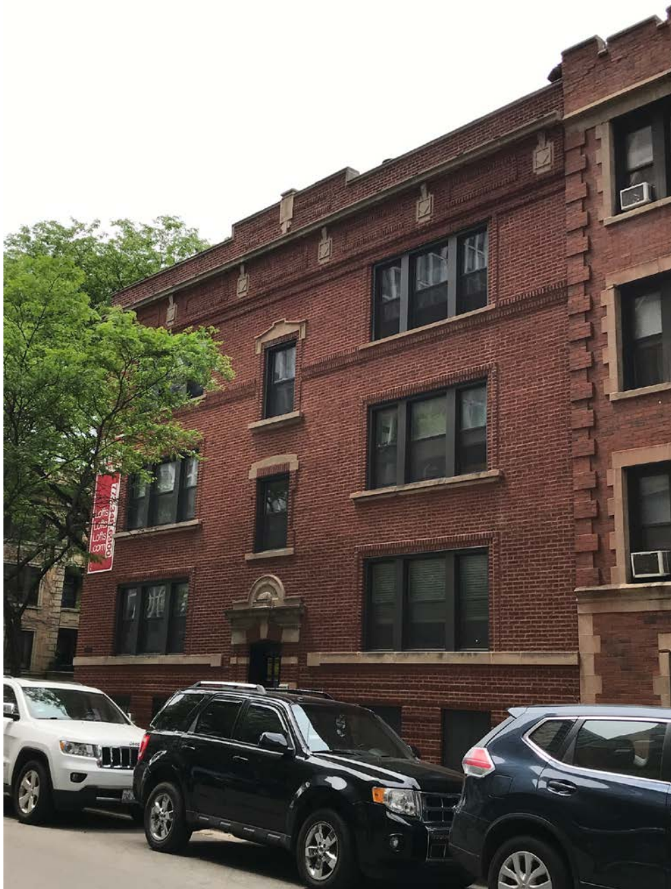
3707-3709 N. Pine Grove Avenue/ 650-652 W. Waveland Avenue, view looking northwest from W. Waveland Avenue toward South façade
