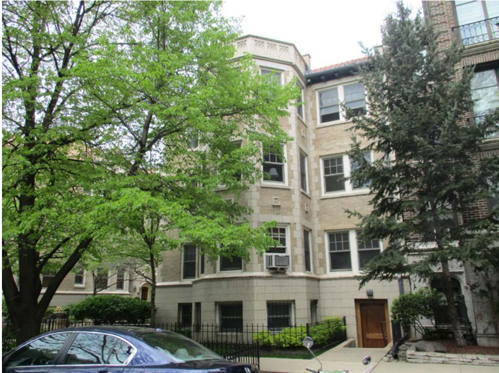
534-552 W. Brompton Avenue, view looking northwest from W. Brompton Avenue toward South façade of East mass
