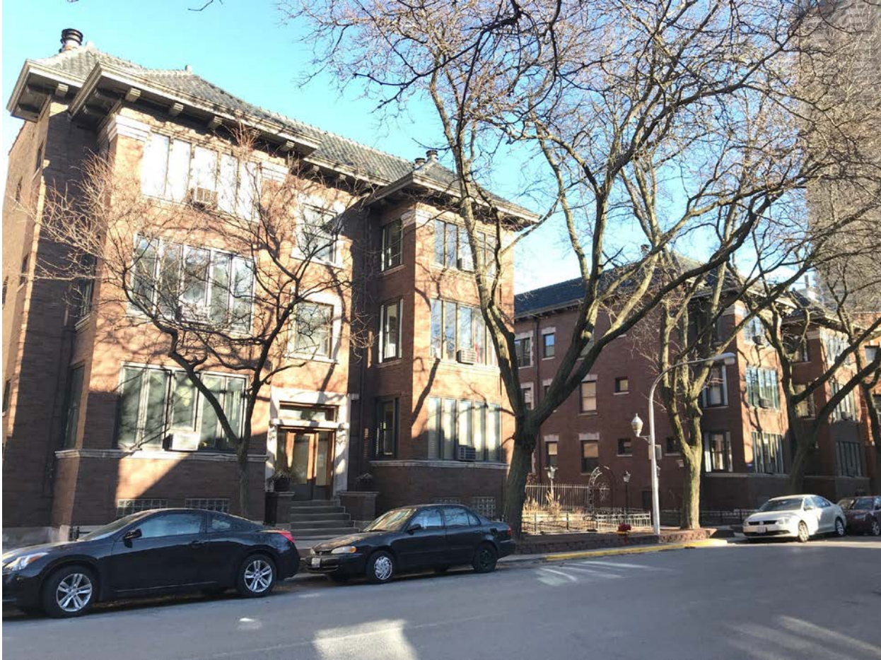
3741-3755 N. Pine Grove Avenue, view looking southeast from N. Pine Grove Avenue toward West façade of North mass and courtyard
