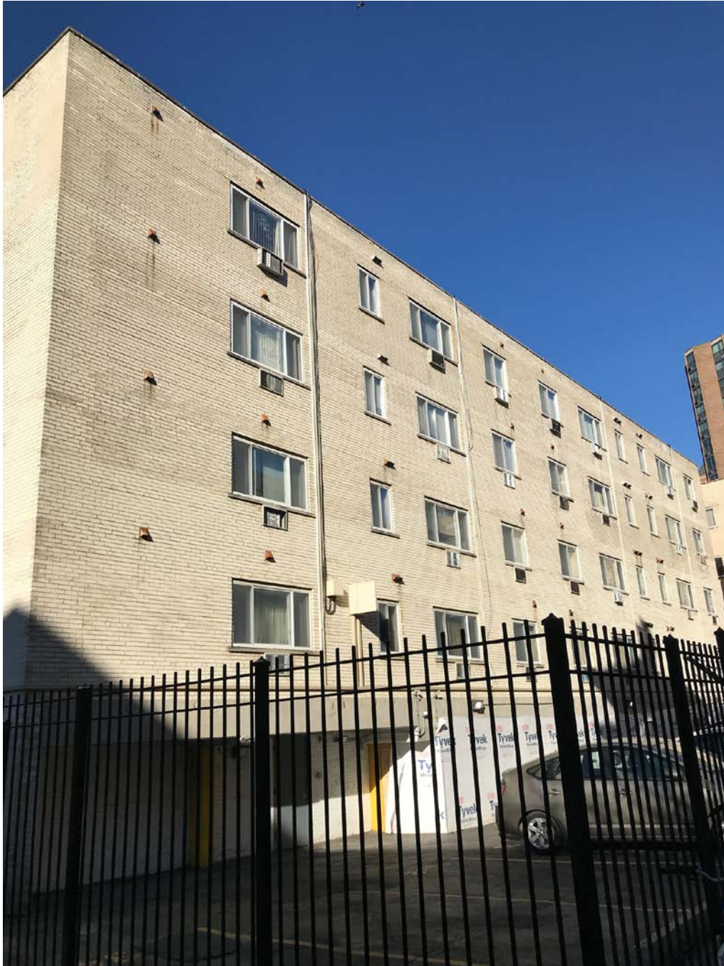
663 W. Grace Street, view looking northeast from N. Pine Grove Avenue toward South façade
