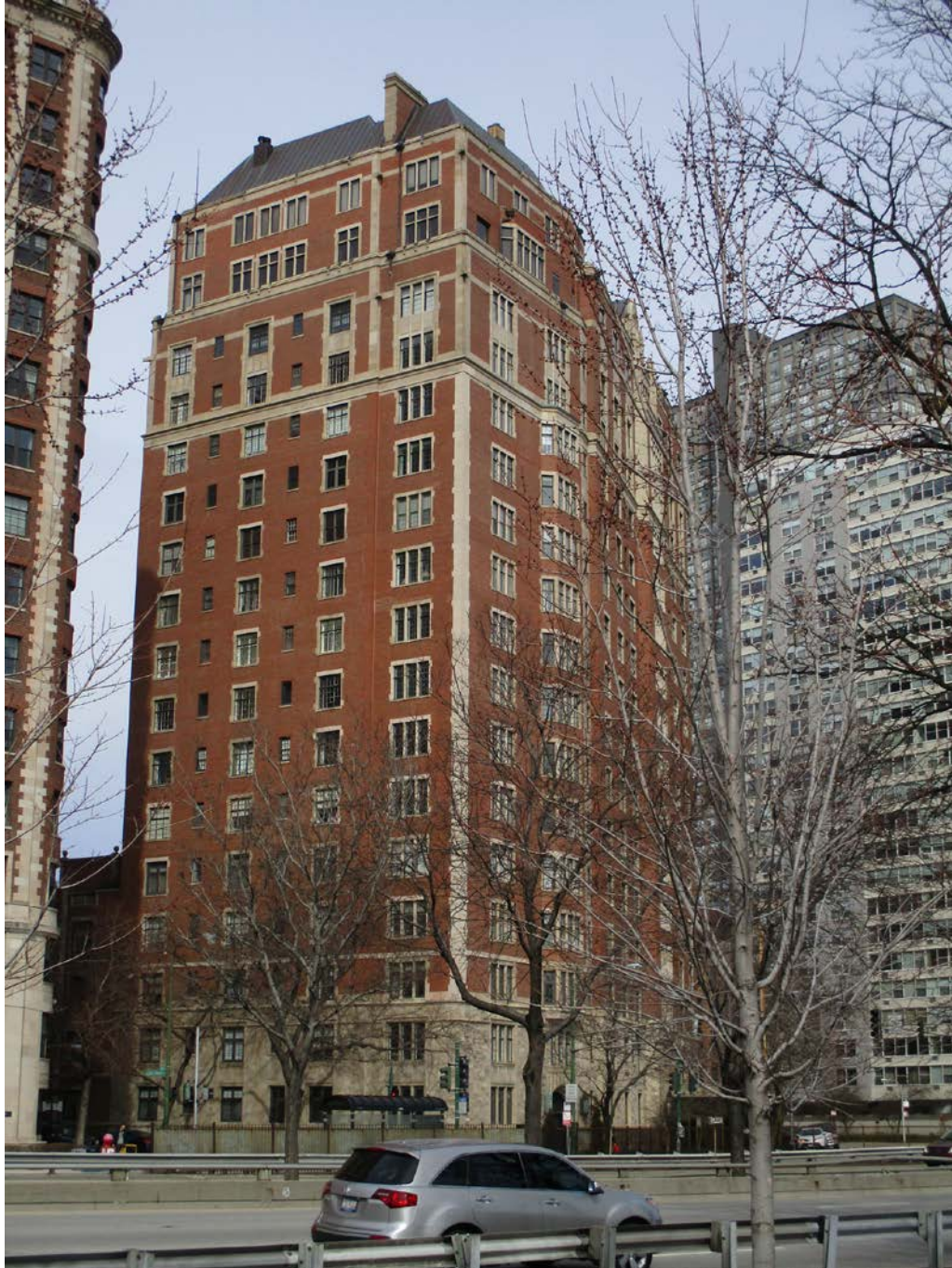
3800 N. Lake Shore Drive, view looking northwest from N. Lake Shore Drive toward South façade
