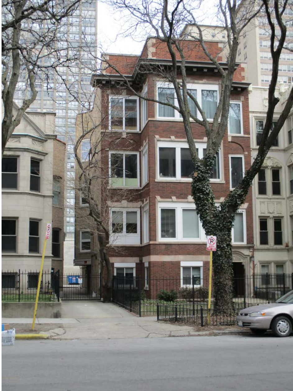
648 W. Sheridan Road, view looking northeast from W. Sheridan Road toward West and South façades
