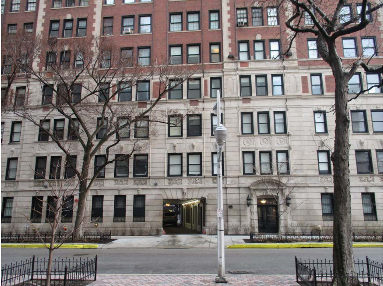
3240 N. Lake Shore Drive, view looking north from W. Melrose Street toward South façade, street level details
