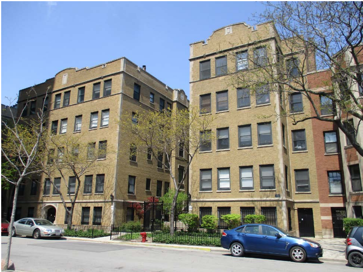
626-640 W. Waveland Avenue, view looking northwest from W. Waveland Avenue toward South façade
