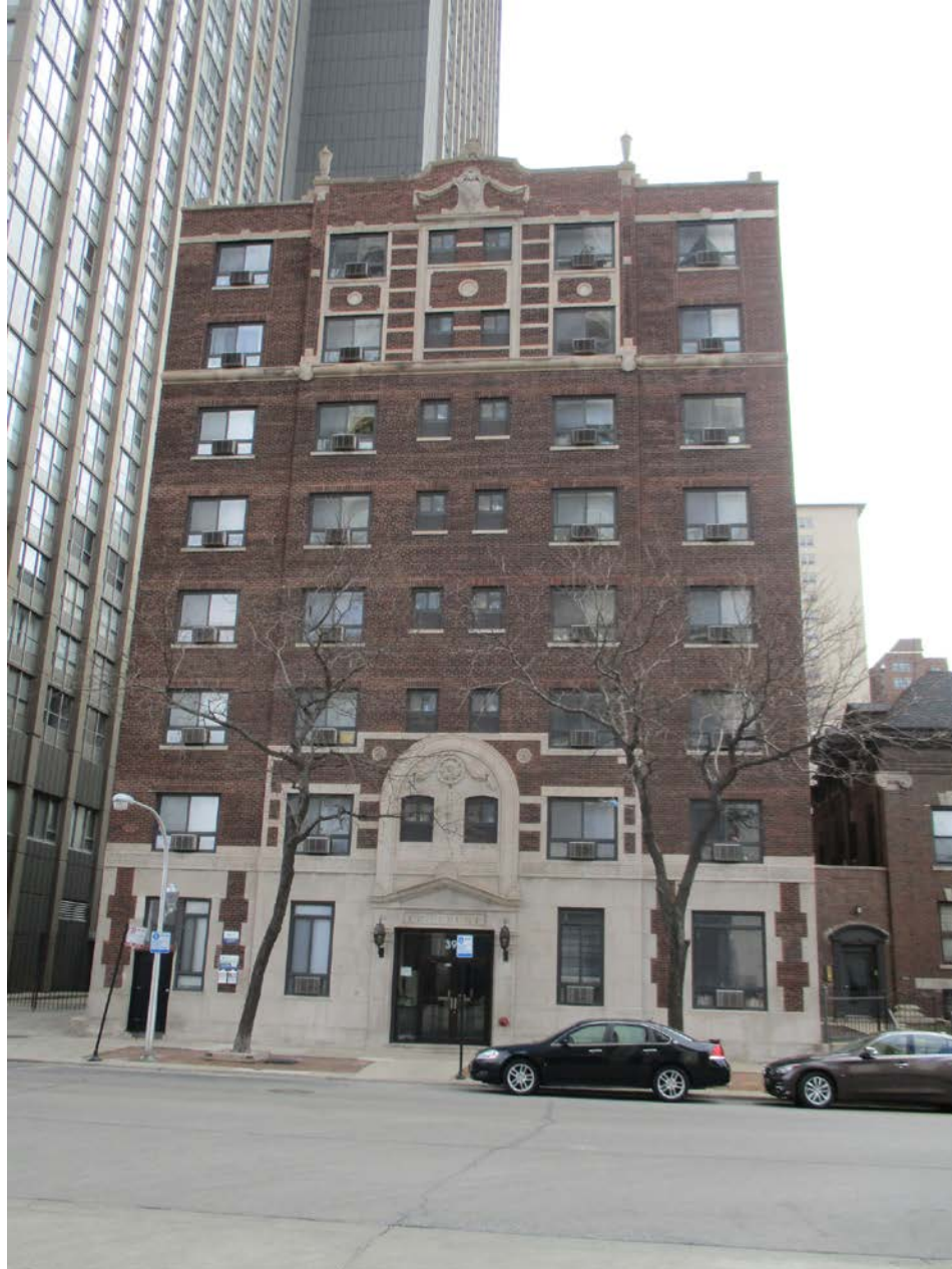
3941 N. Pine Grove Avenue, view looking east from N. Pine Grove Avenue toward West façade
