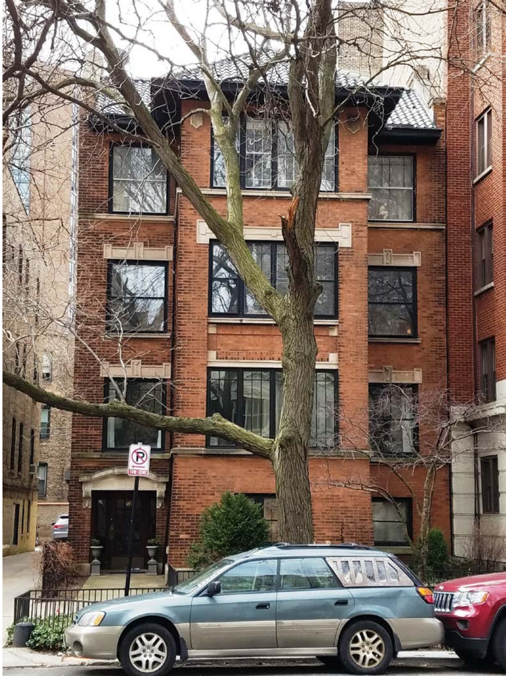
645 W. Sheridan Road, view looking south from W. Sheridan Road toward North façade
