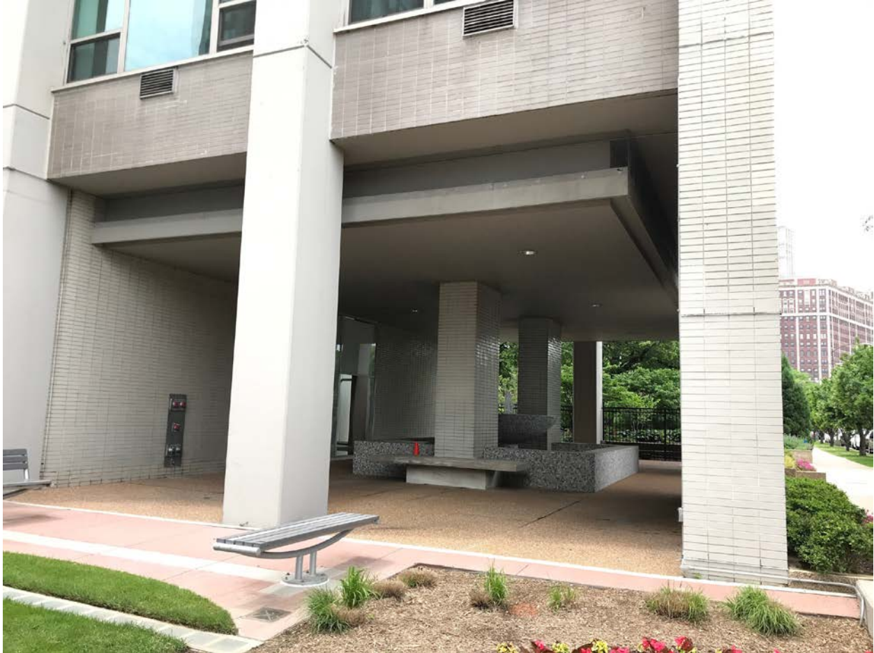
3600 N. Lake Shore Drive, view looking northwest from driveway toward base-level atrium of North tower
