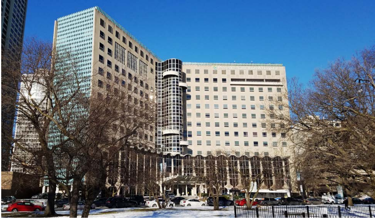
2900 N. Lake Shore Drive, view looking west from N. Lake Shore Drive toward East façade (front entrance)
