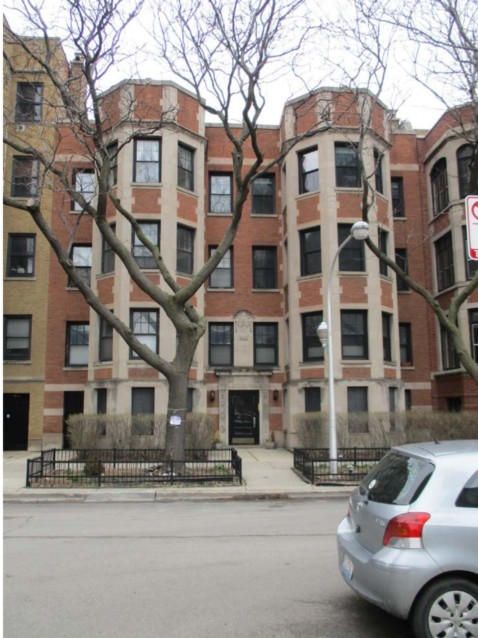
620-622 W. Waveland Avenue, view looking north from W. Waveland Avenue toward South façade
