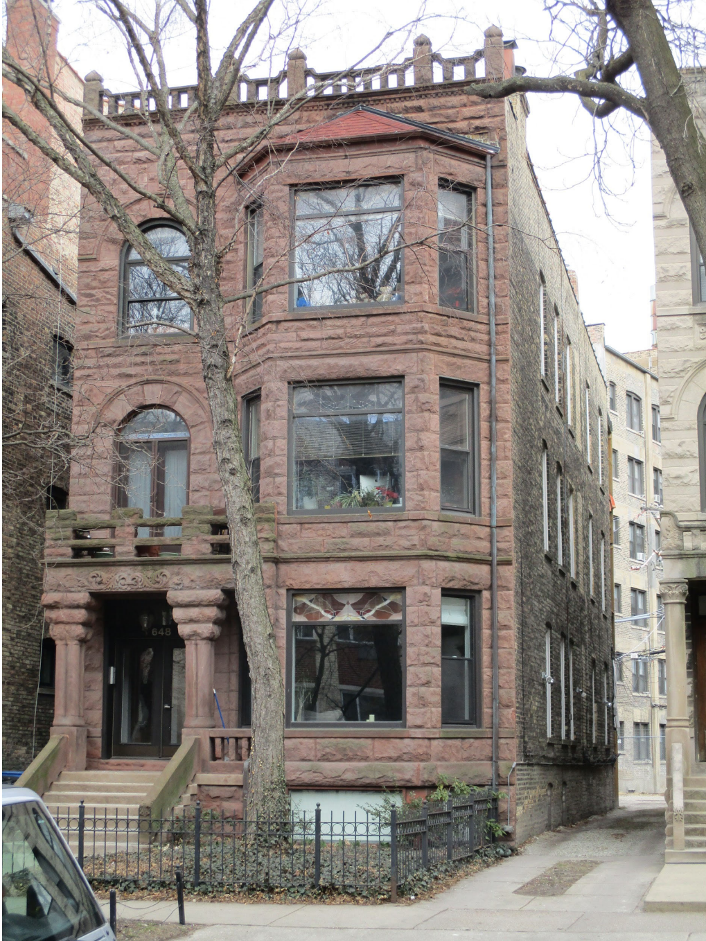
648 W. Grace Street, view looking northwest from W. Grace Street toward South and East façades
