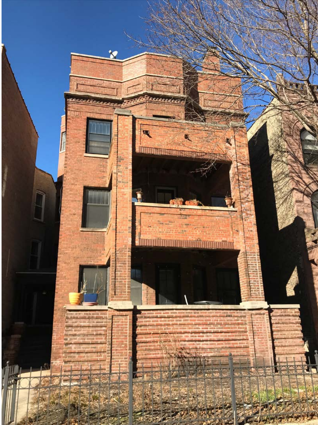
650 W. Grace Street, view looking northeast from W. Grace Street toward South façade
