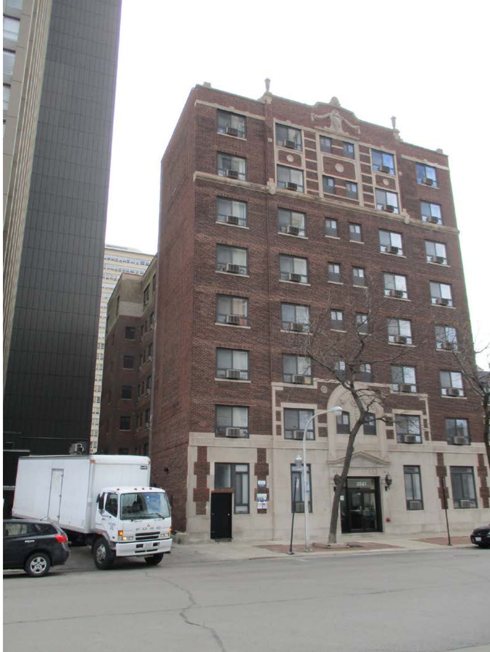
3941 N. Pine Grove Avenue, view looking southeast from N. Pine Grove Avenue toward North and West façades
