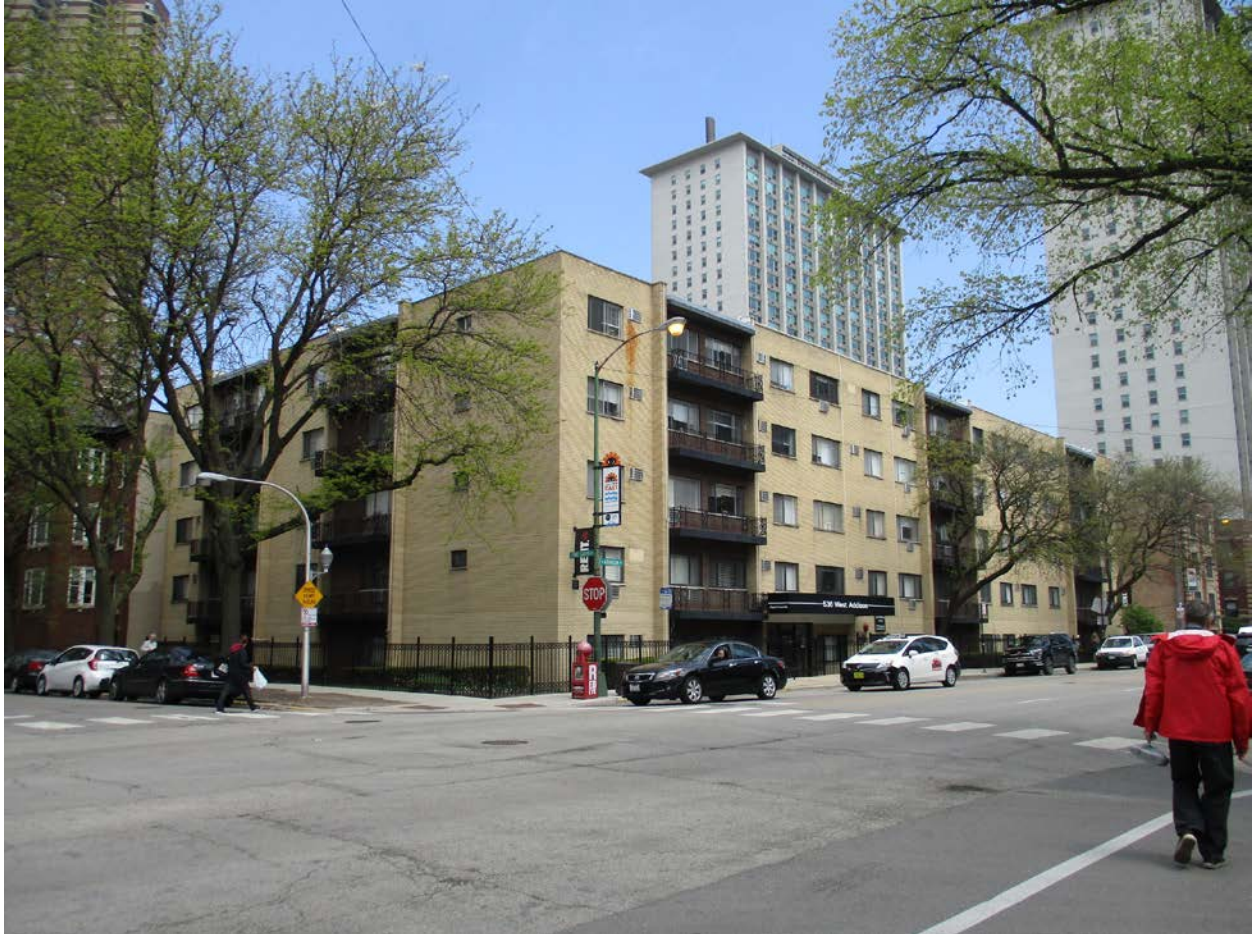
536 W. Addison Street, view looking northeast from intersection of W. Addison Street and N. Pine Grove Avenue toward West and South façades
