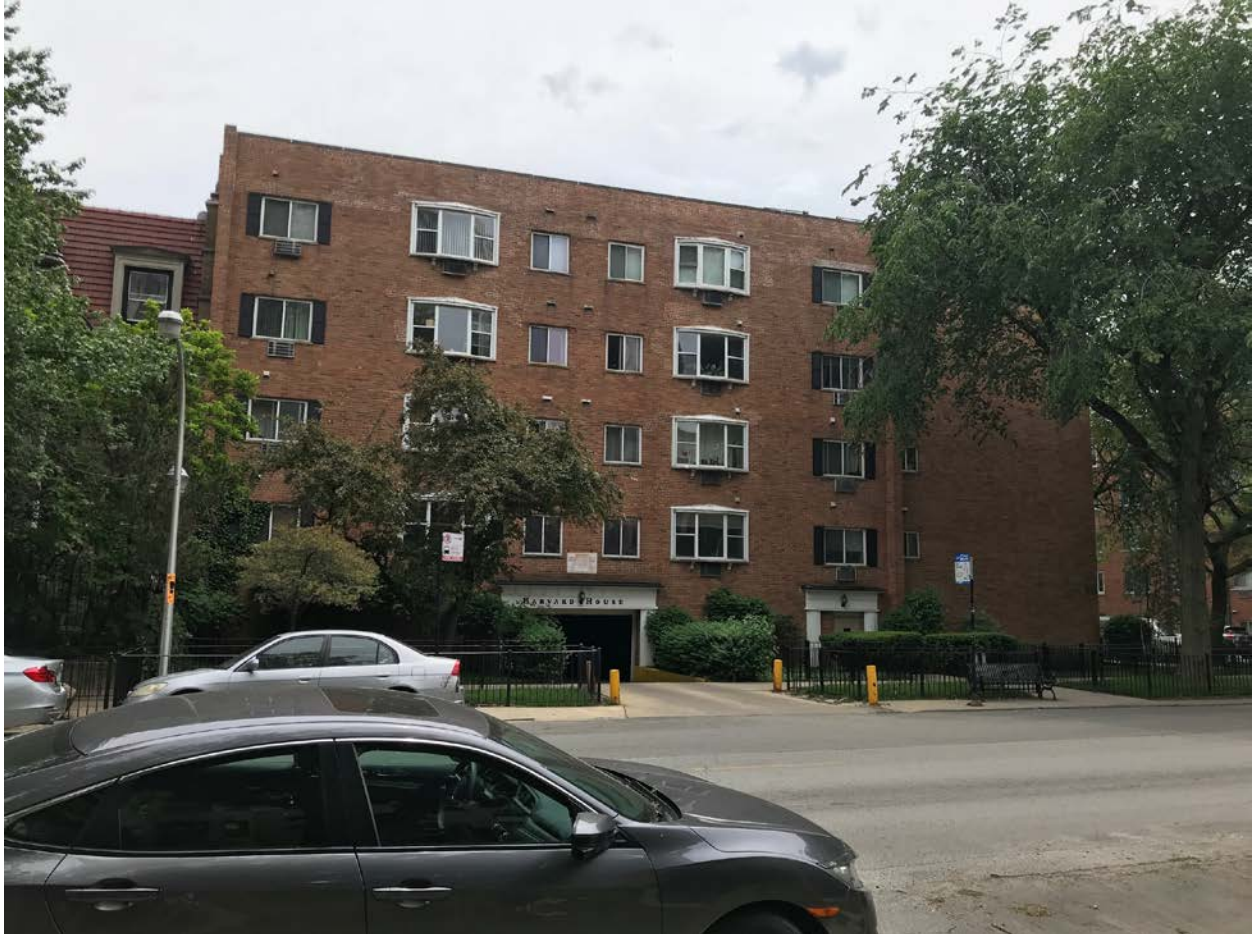
3825 N. Pine Grove Avenue, view looking southwest from W. Sheridan Road toward North façade
