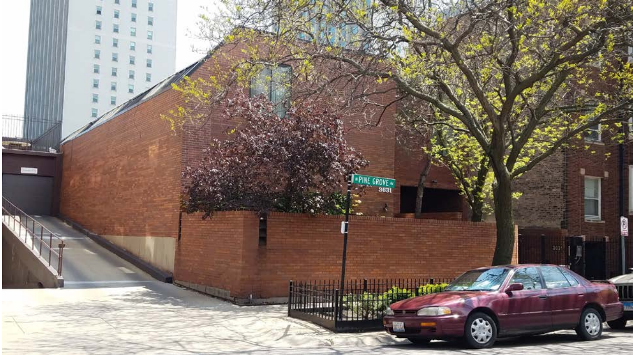
3631 N. Pine Grove Avenue, view looking southeast from N. Pine Grove Avenue toward North and West façades
