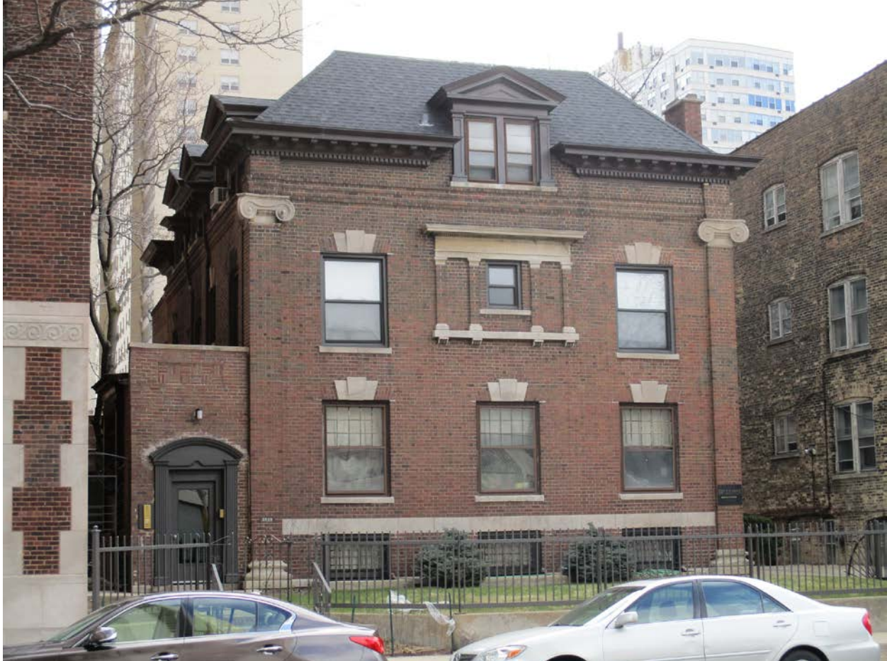
3939 N. Pine Grove Avenue, view looking southeast from N. Pine Grove Avenue toward North and West façades
