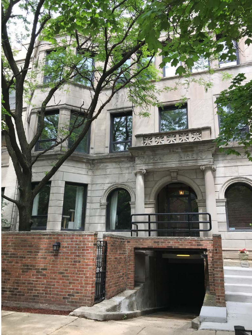
3717-3719 N. Pine Grove Avenue, view looking northeast from N. Pine Grove Avenue toward West façade
