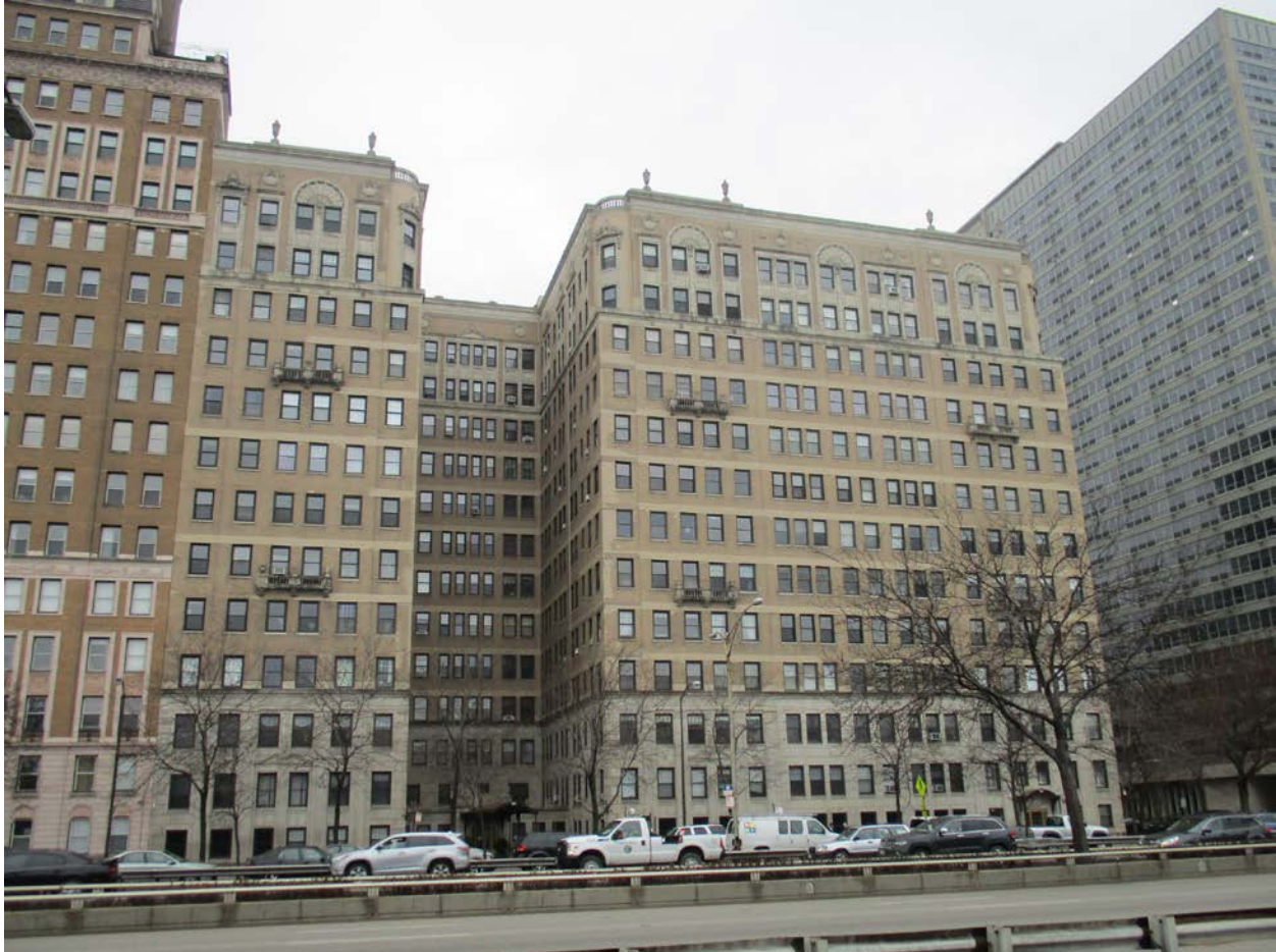
3520-3530 N. Lake Shore Drive, view looking northwest from N. Lake Shore Drive toward East façade and South courtyard facade
