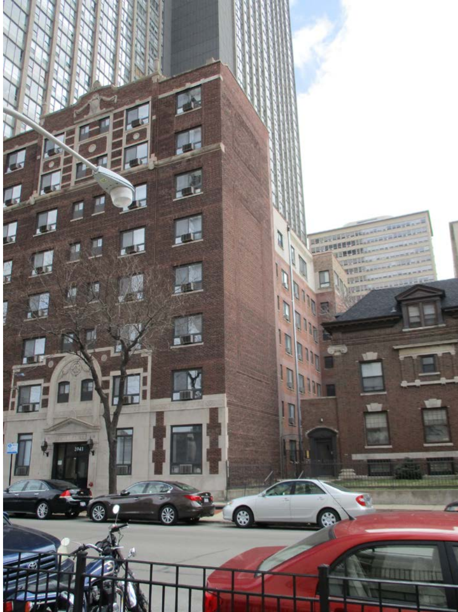
3941 N. Pine Grove Avenue, view looking northeast from N. Pine Grove Avenue toward West and South façades
