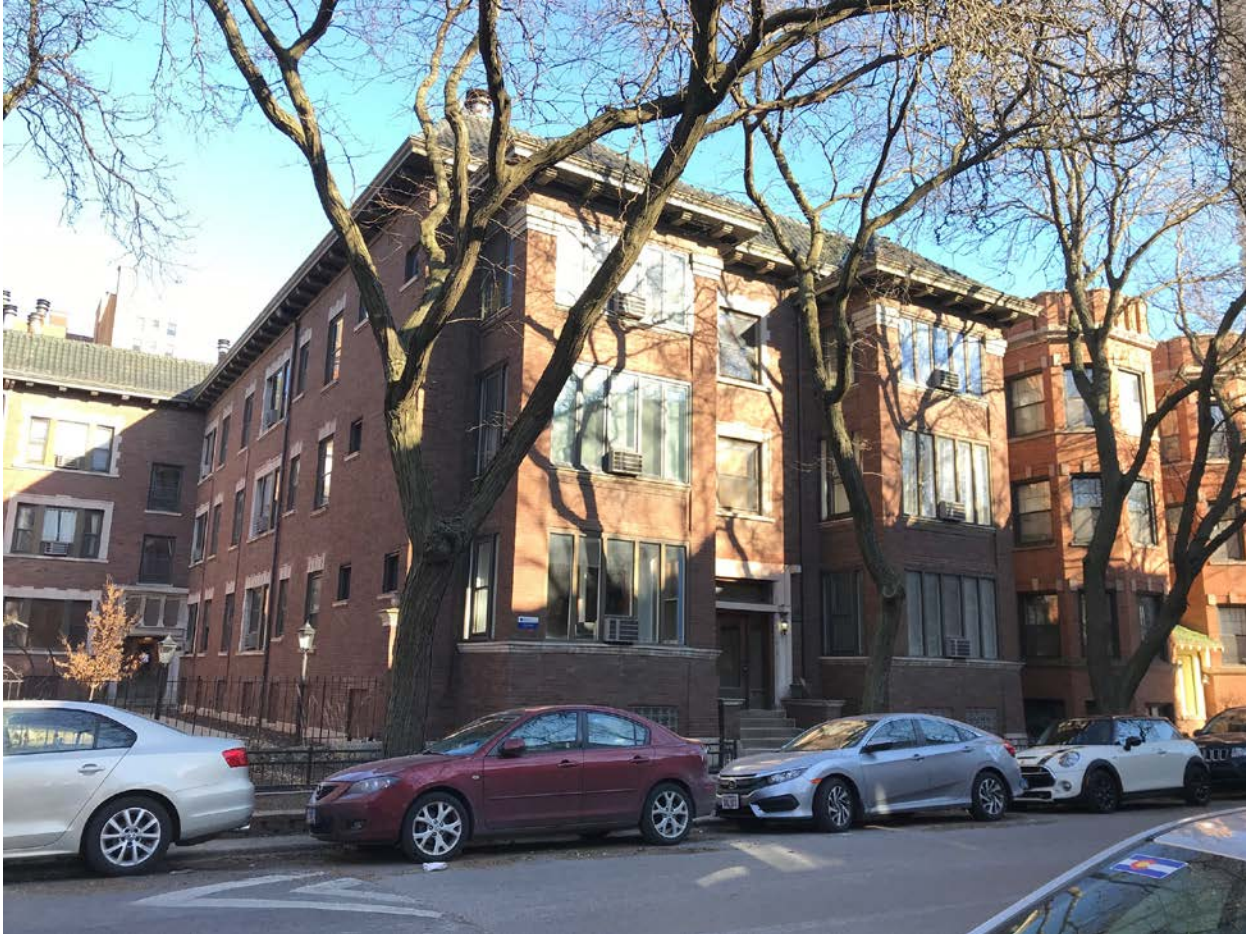
3741-3755 N. Pine Grove Avenue, view looking southeast from N. Pine Grove Avenue toward North and West façades of South mass
