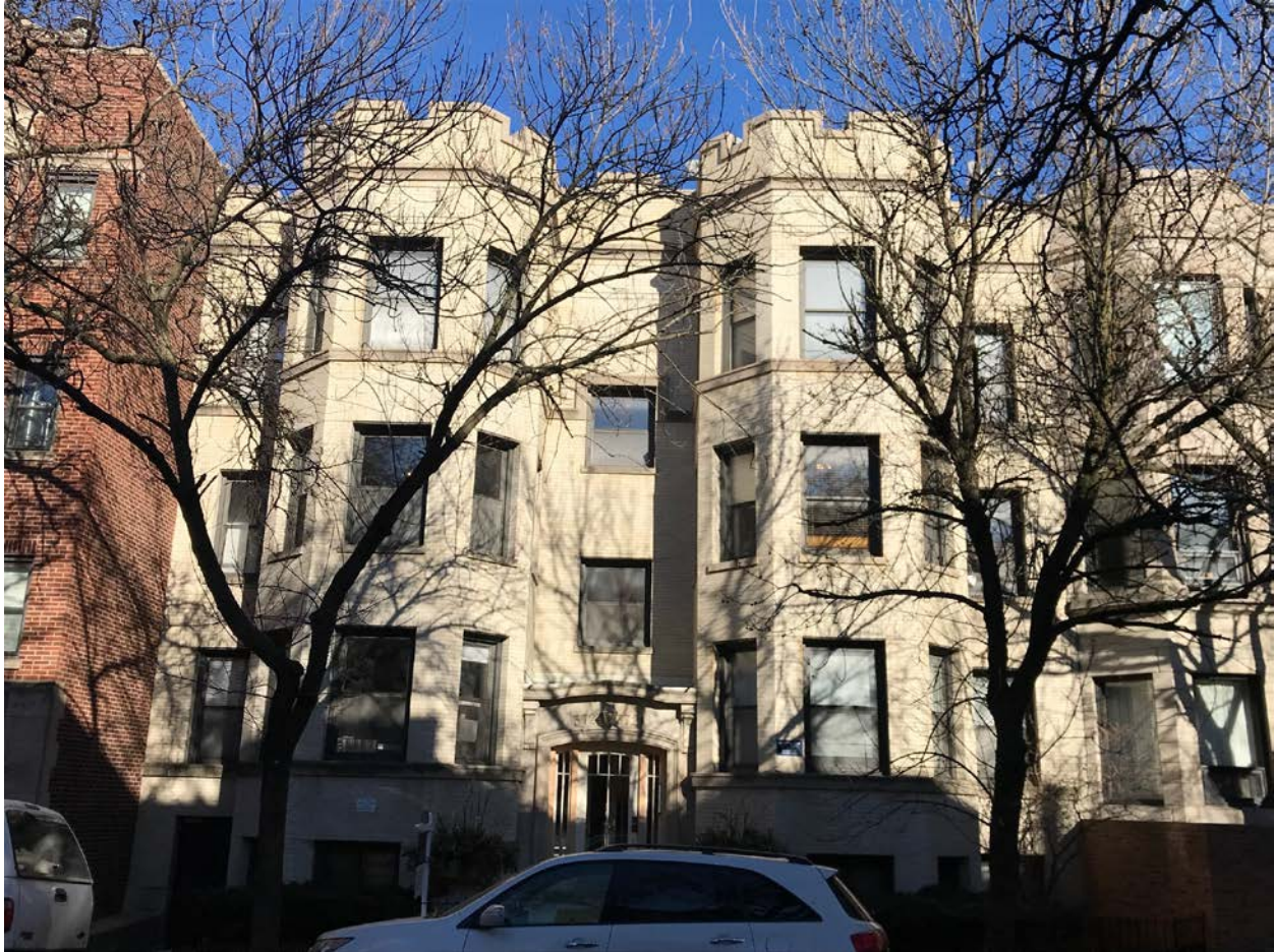
3721-23 N. Pine Grove Avenue, view looking east from N. Pine Grove Avenue toward West façade
