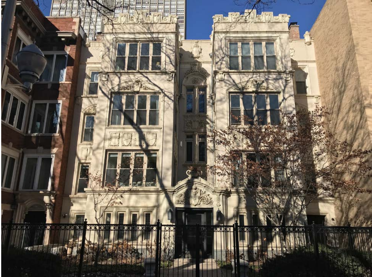
644-646 W. Sheridan Road, view looking north from W. Sheridan Road toward South façade
