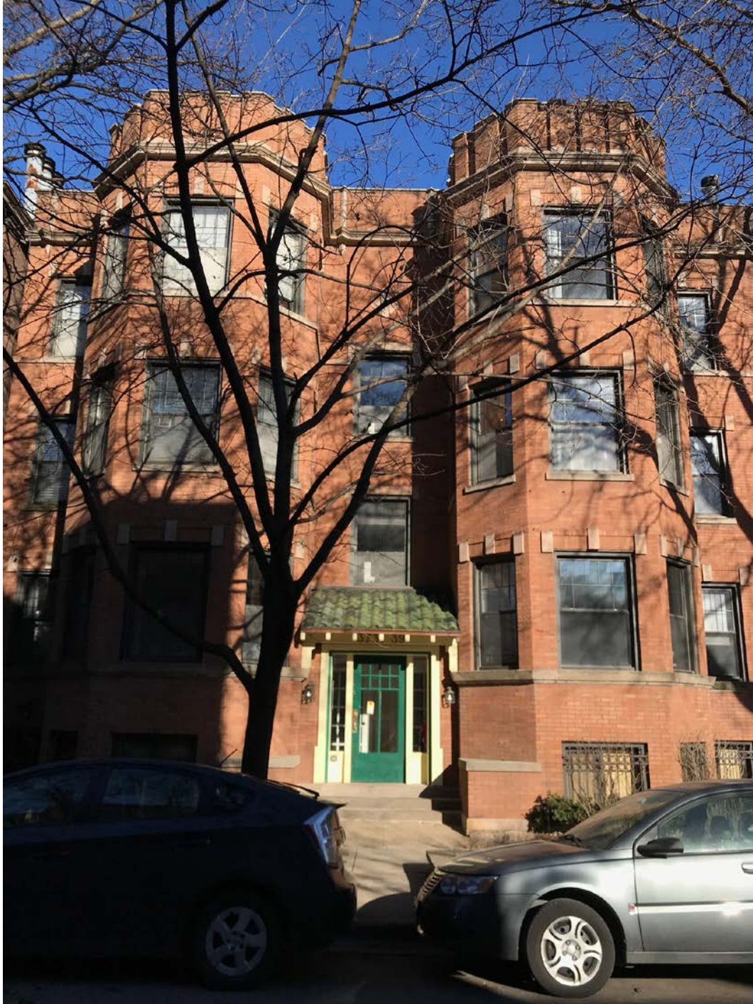
3737-3739 N. Pine Grove Avenue, view looking east from N. Pine Grove Avenue toward West façade
