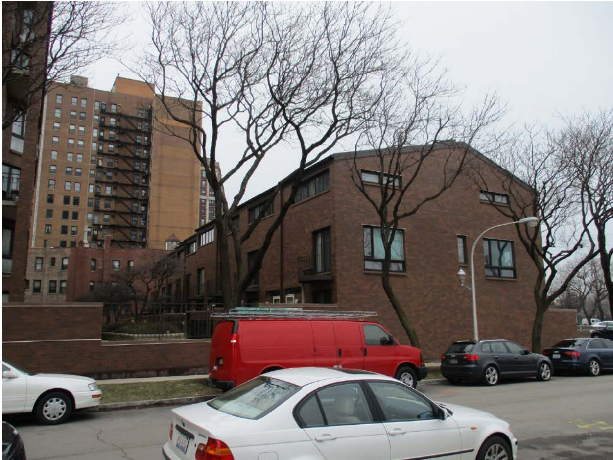
3700 N. Lake Shore Drive, view looking northeast from W. Waveland Avenue toward South and West facades.
