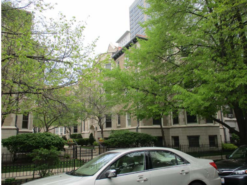
534-552 W. Brompton Avenue, view looking northeast from W. Brompton Avenue toward East courtyard
