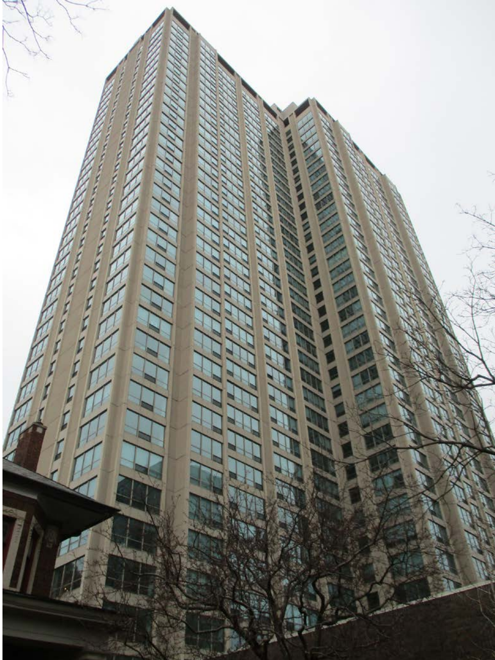
3450 N. Lake Shore Drive, view looking northeast from W. Hawthorne Place toward West and South façades
