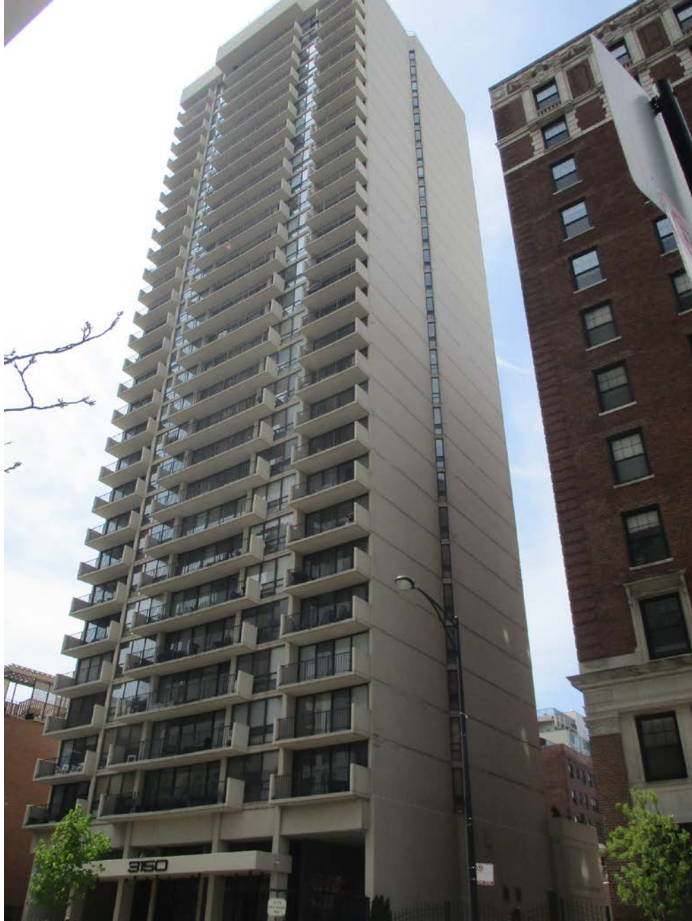
3150 N. Sheridan Road, view looking southwest from N. Sheridan Road toward East and North façades
