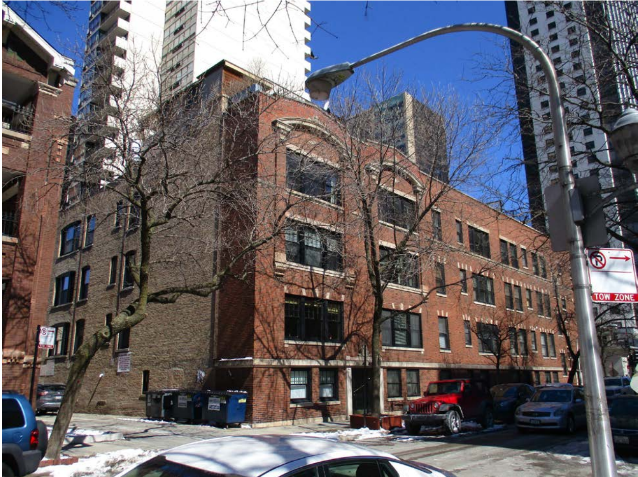
3140-3144 N. Sheridan Road/ 400-410 W. Briar Place, view looking northeast from W. Briar Place toward West and South façades
