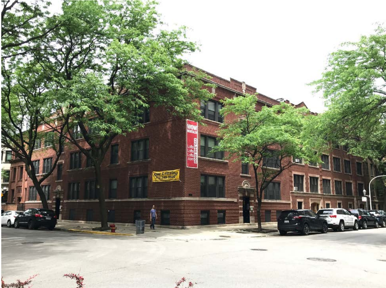
3707-3709 N. Pine Grove Avenue/ 650-652 W. Waveland Avenue, view looking northeast from intersection of N. Pine Grove Avenue and W. Waveland Avenue toward West and South façades
