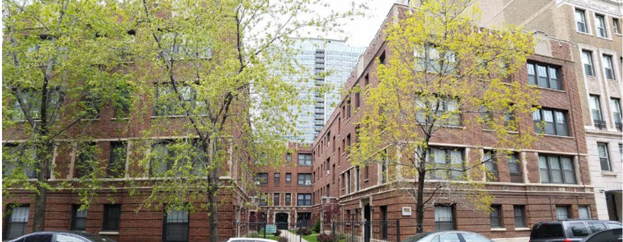
512-520 W. Cornelia Avenue, view looking north from W. Cornelia Avenue toward courtyard and South façades
