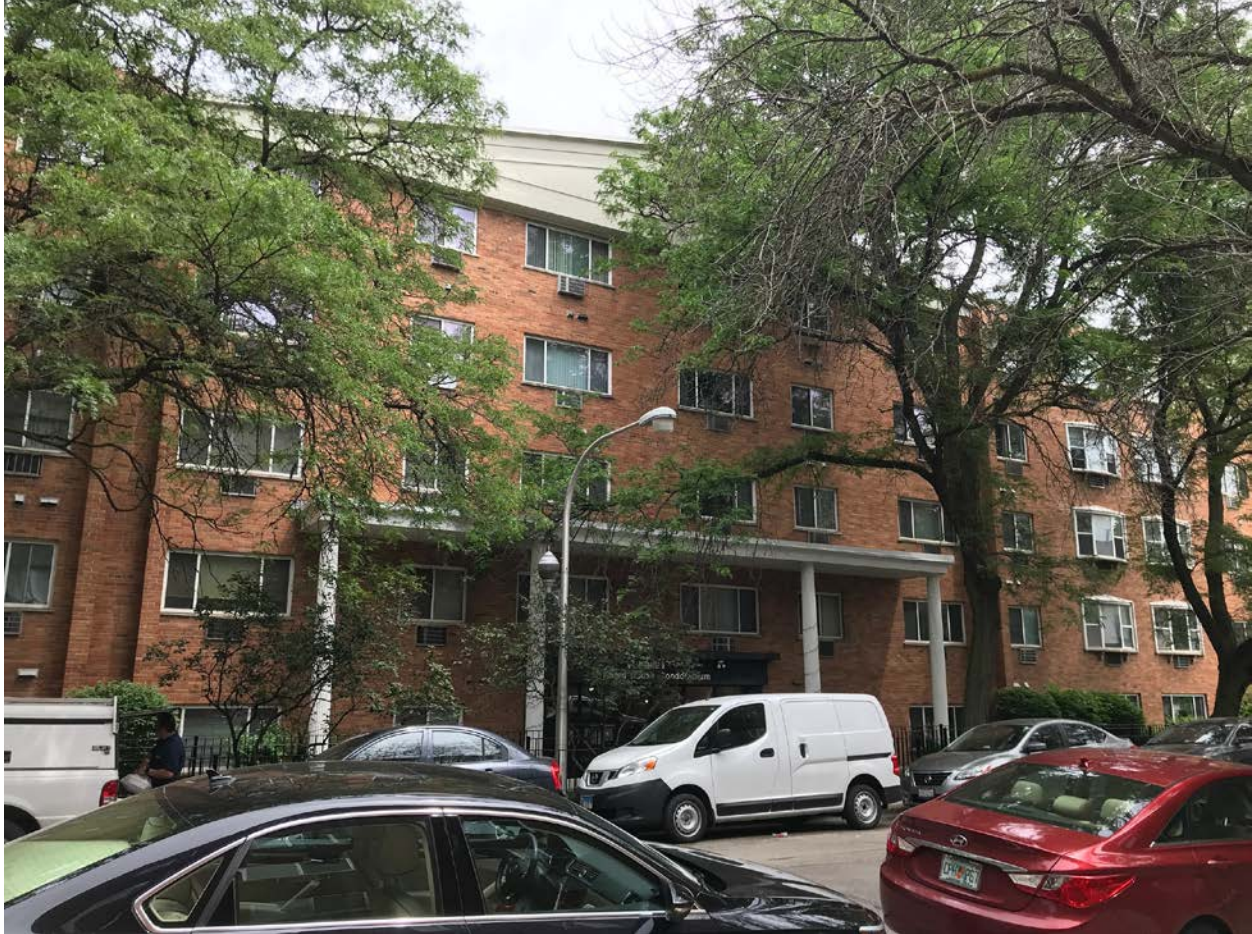
3825 N. Pine Grove Avenue, view looking southeast from N. Pine Grove Avenue toward West façade
