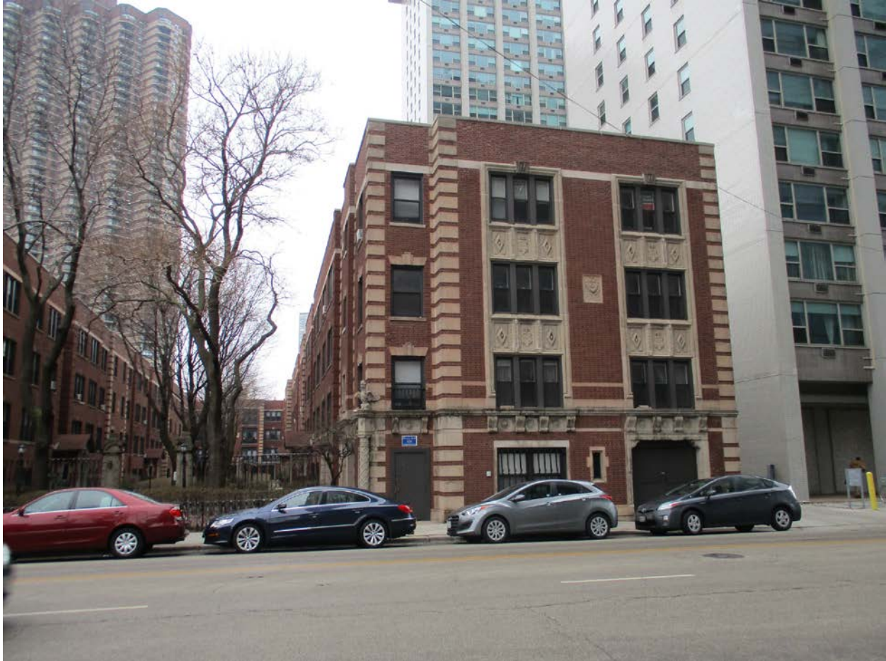
512 ½ - 534 ½ W. Addison Street, view looking north from W. Addison Street toward South façade of East mass
