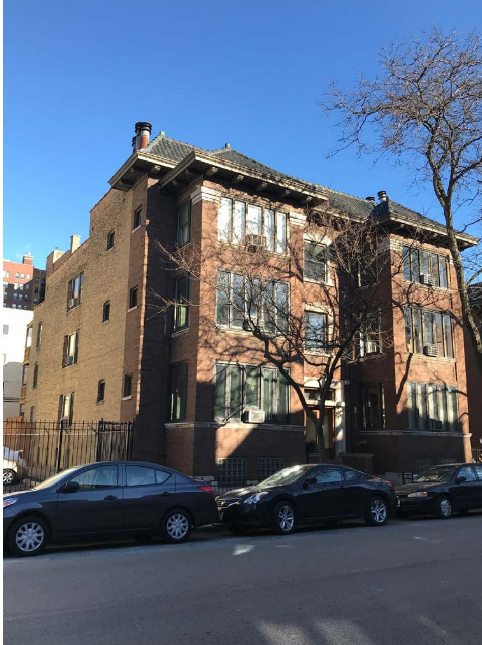
3741-3755 N. Pine Grove Avenue, view looking southeast from N. Pine Grove Avenue toward North and West façades of North mass
