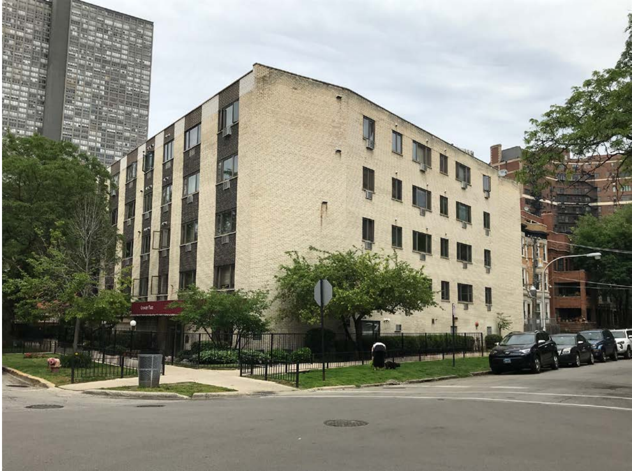
3801 N. Pine Grove Avenue, view looking northeast from N. Pine Grove Avenue toward South façade
