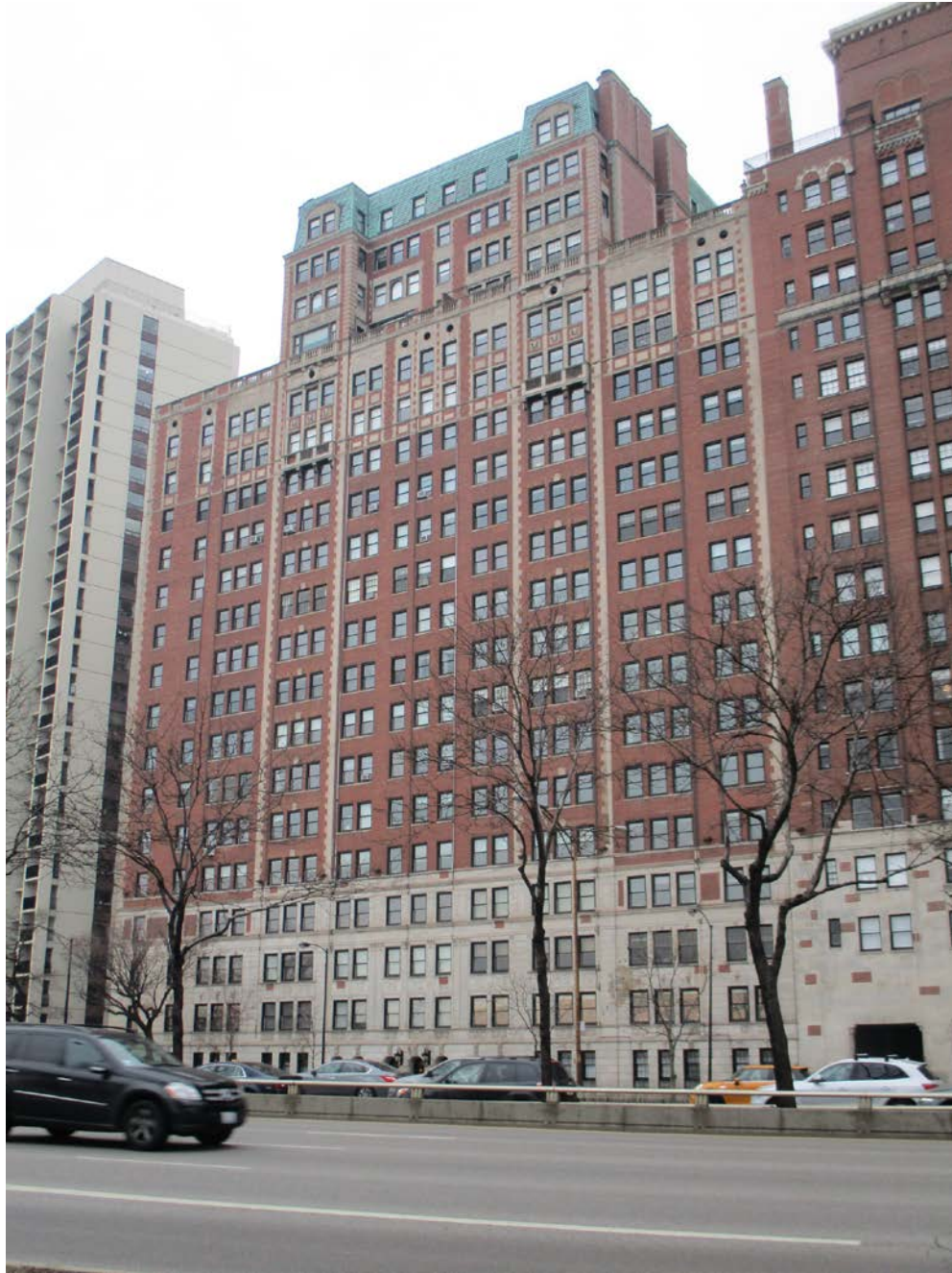
3260-3270 N. Lake Shore Drive, view looking southwest from N. Lake Shore Drive toward East façade
