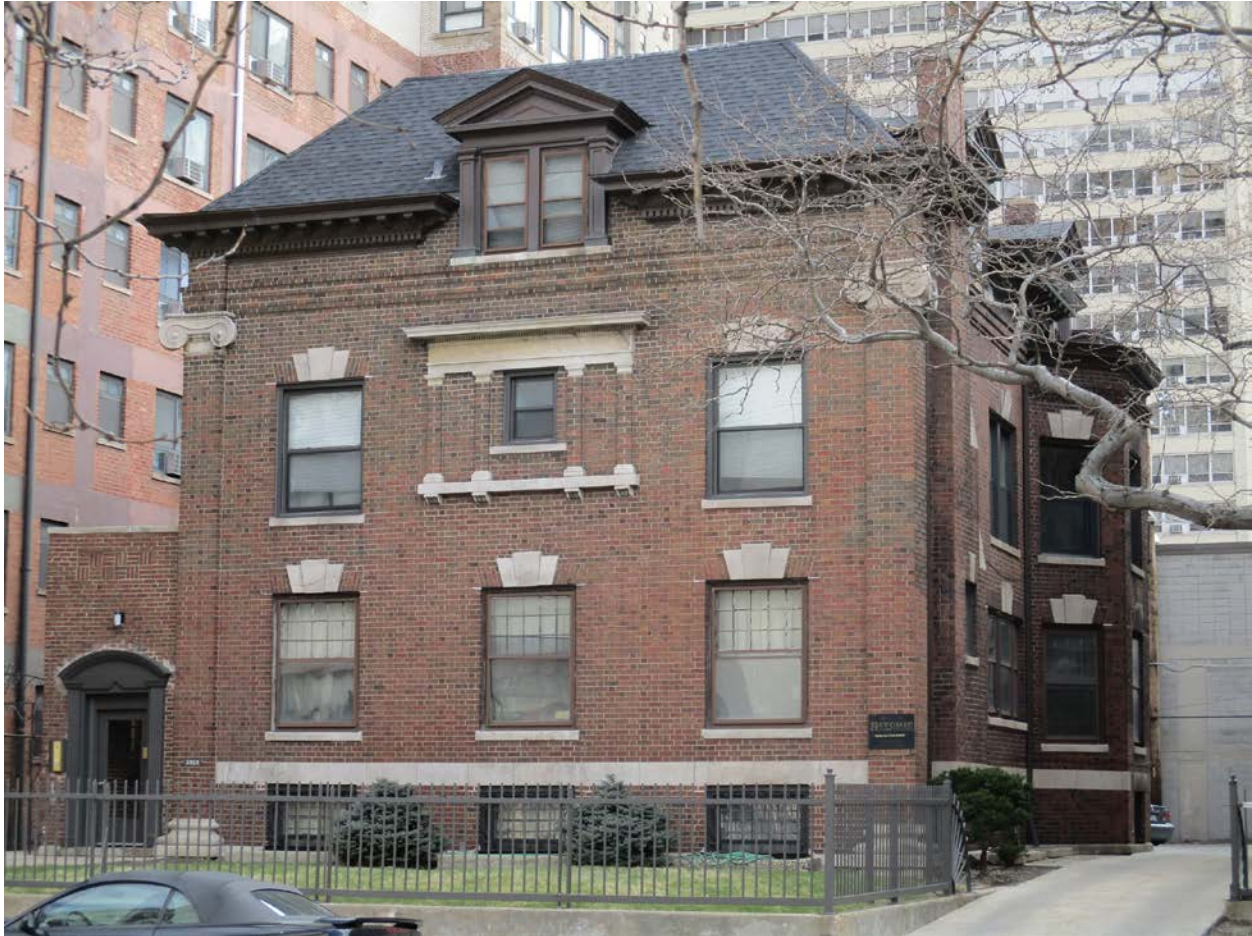
3939 N. Pine Grove Avenue, view looking northeast from N. Pine Grove Avenue toward West and South façades
