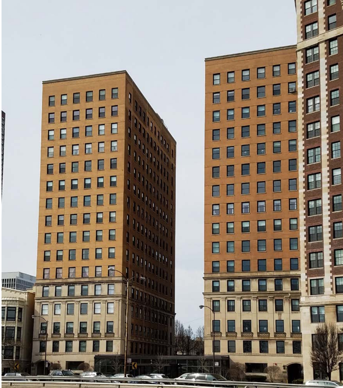
3730-3740 N. Lake Shore Drive, view looking southwest from N. Lake Shore Drive toward East façades and North facade of South tower
