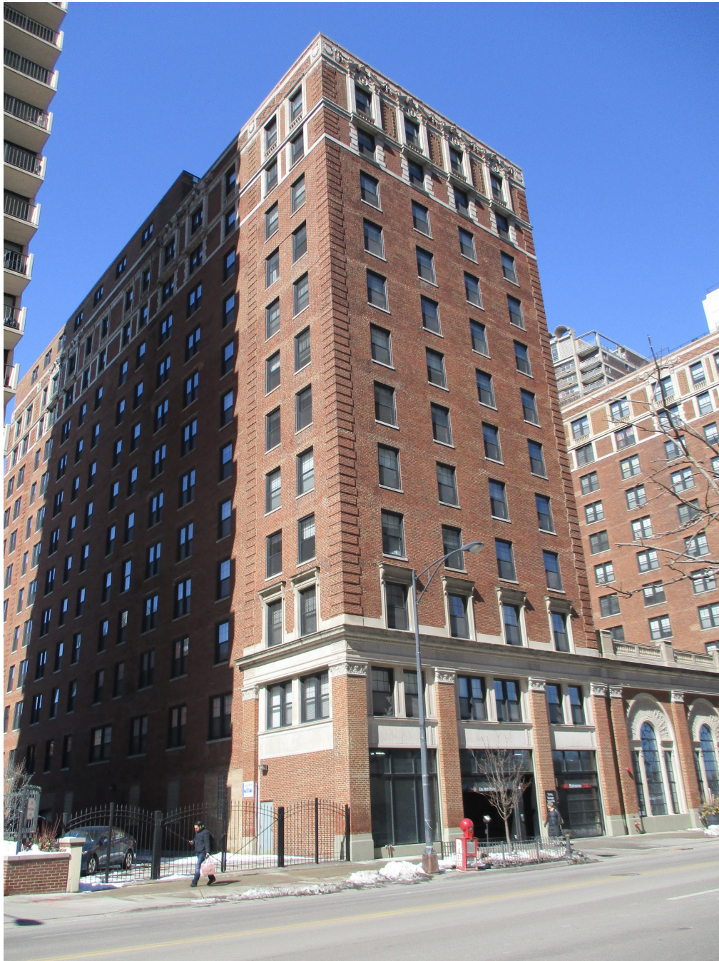
3170 N. Sheridan Road, view looking northwest from N. Sheridan Road toward South and East façades
