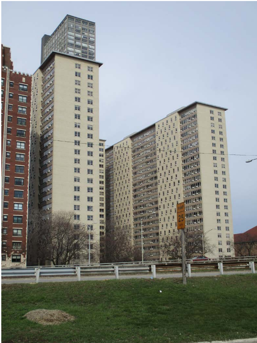
3950 N. Lake Shore Drive, view looking northwest from N. Lake Shore Drive toward East and South façades
