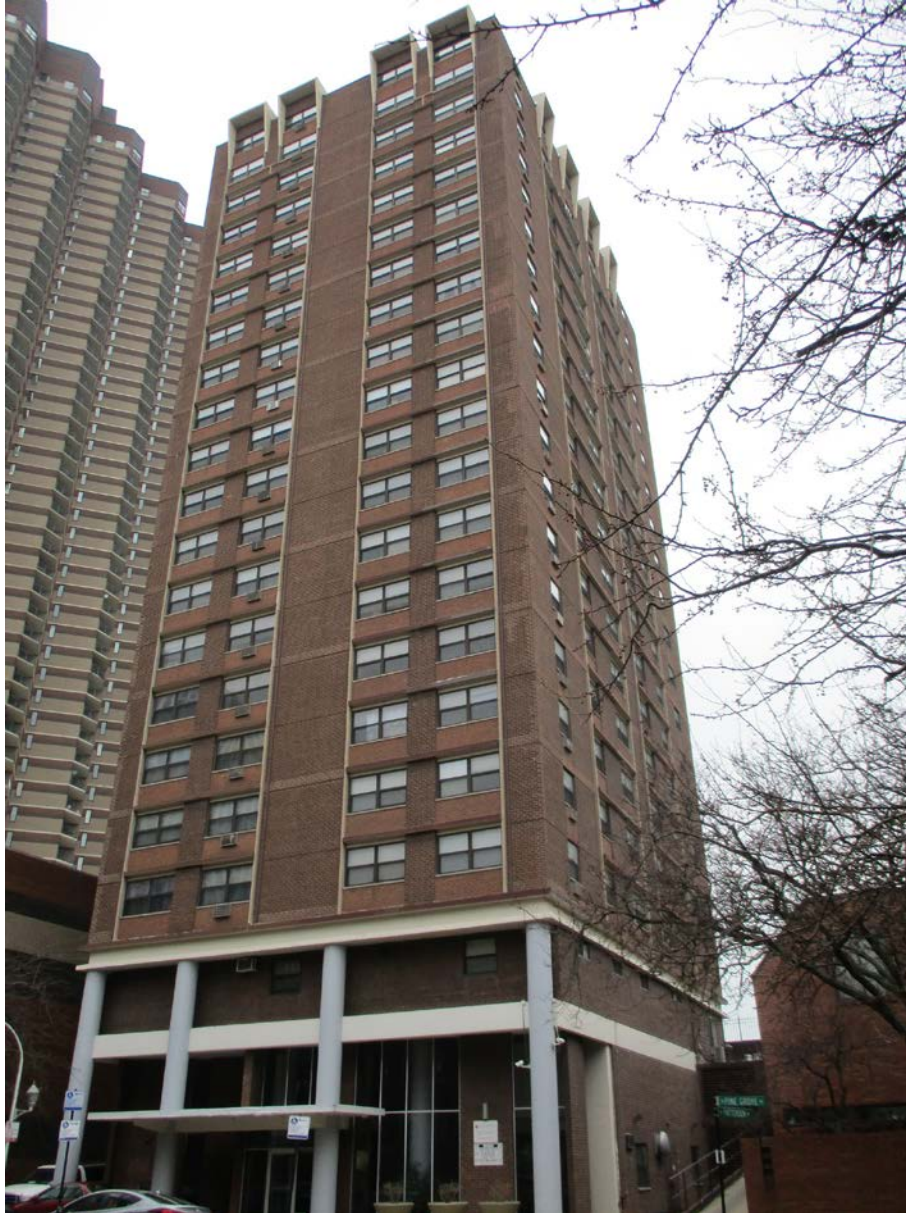
3639 N. Pine Grove Avenue, view looking northeast from N. Pine Grove Avenue toward West and South façades
