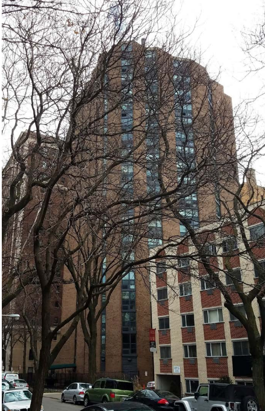
635 W. Grace Street, view looking southeast from W. Grace Street toward West façade
