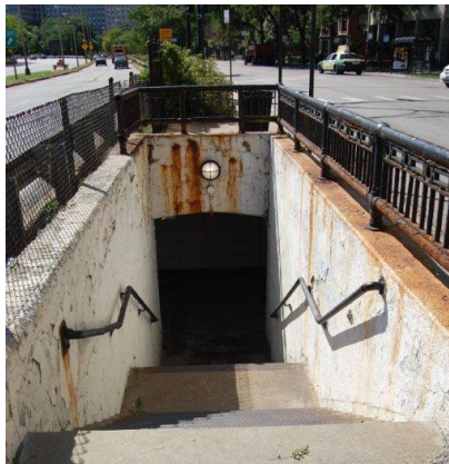
Exhibit 2-4: Existing Pedestrian Underpass
