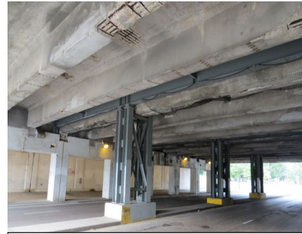
Exhibit 2-3: Temporary Bridge Supports
