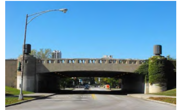
Fullerton LSD Bridge, 1941
