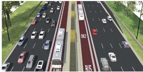
The Addition (Dedicated Transitway-Left)
