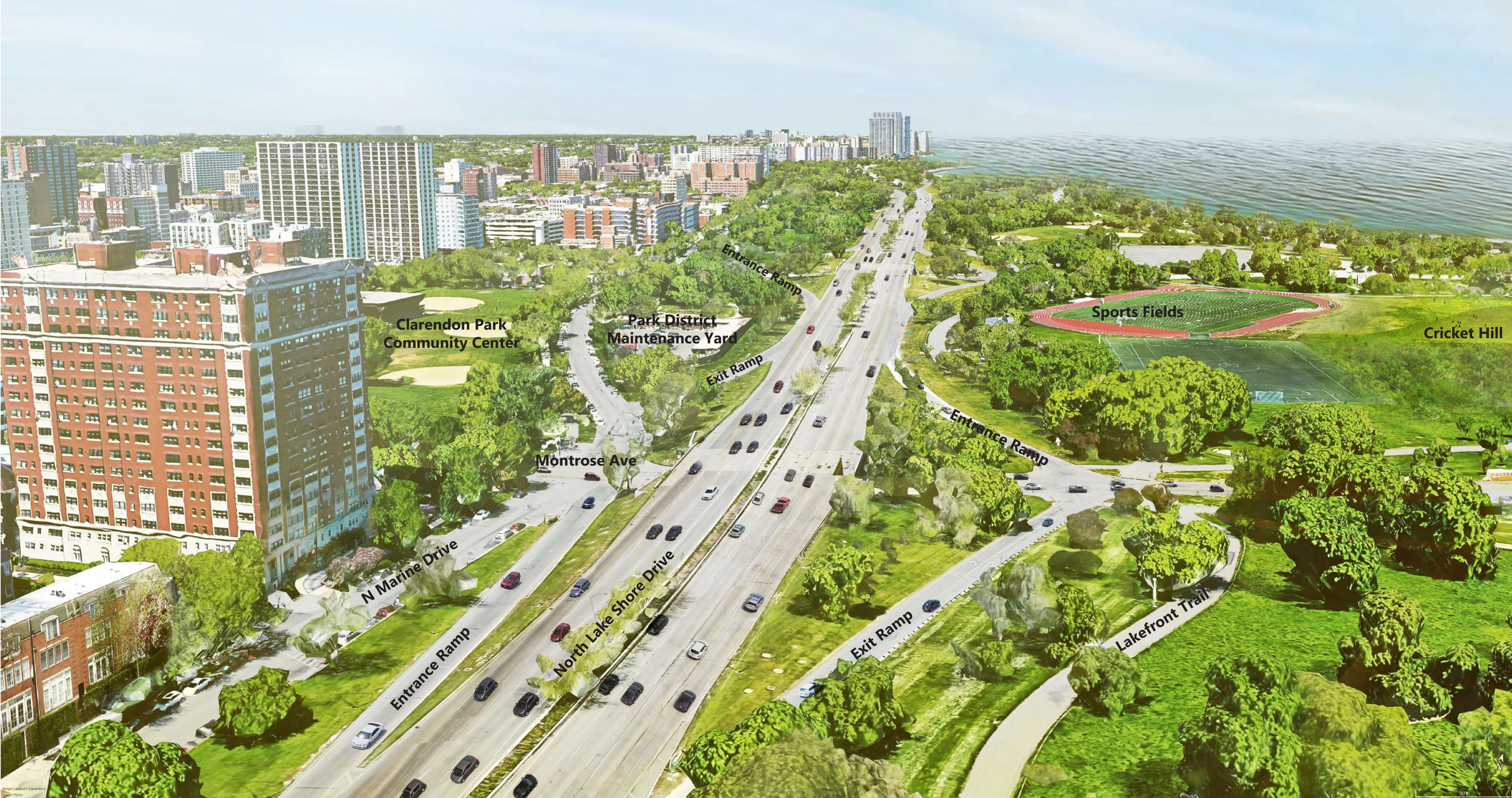
Montrose Ave Junction Looking North - EXISTING VIEW
