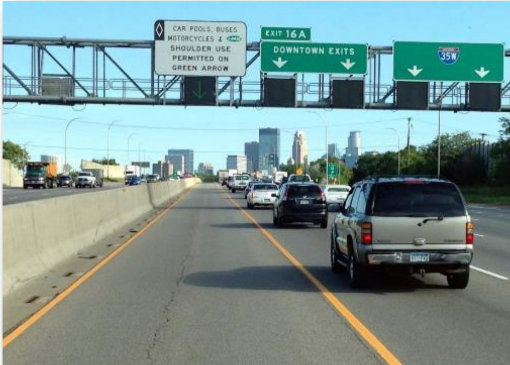
I-35 Multi-Purpose Lane (Minneapolis, MN)
