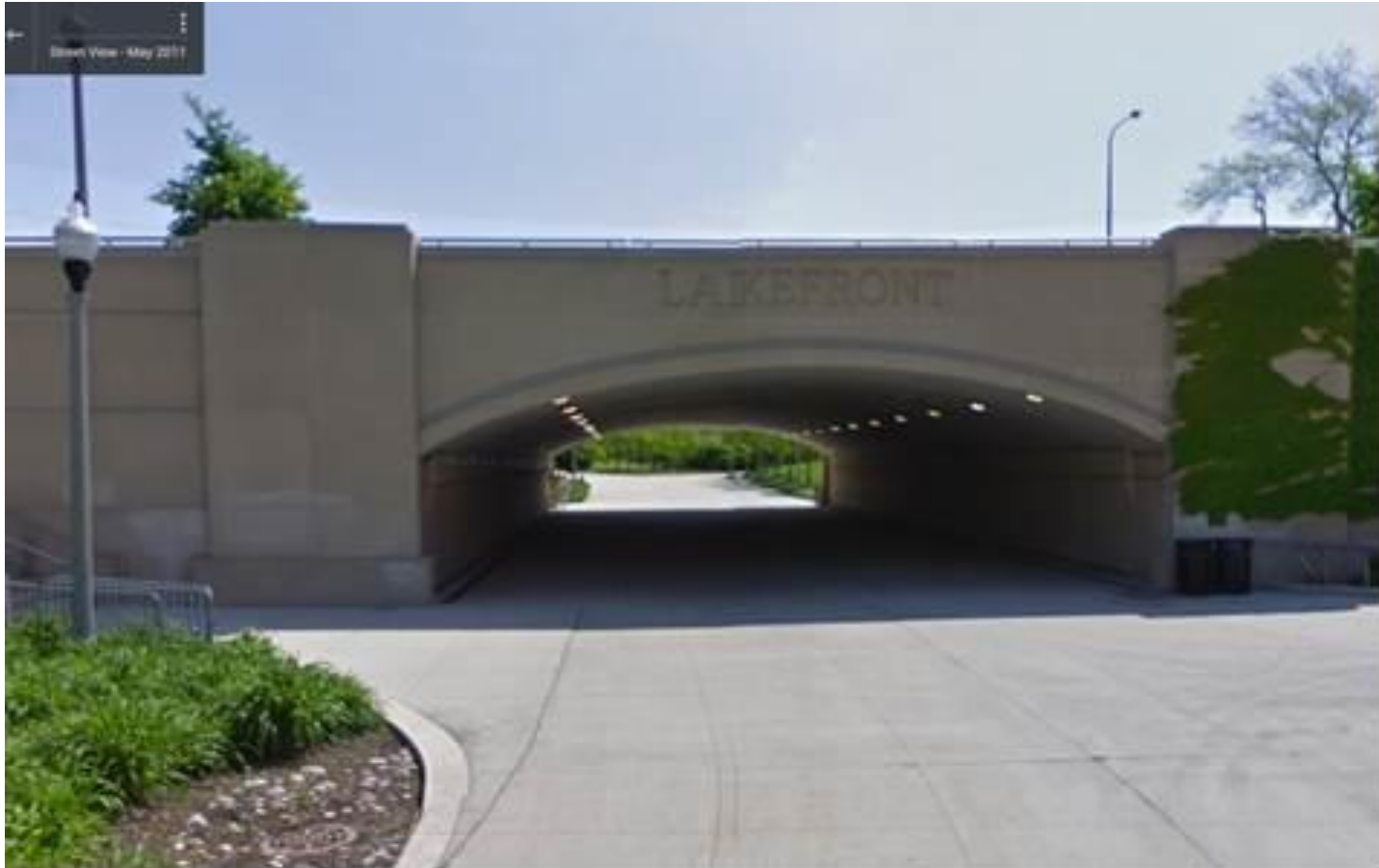
Example Underpass Grant Park
