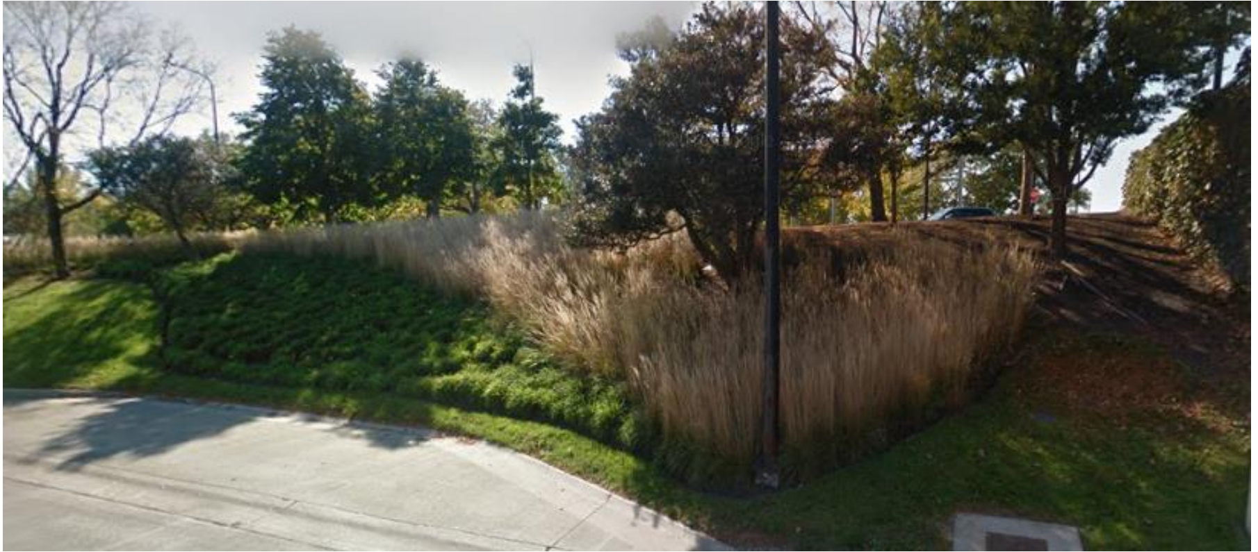
Example Embankment South Lake Shore Drive
